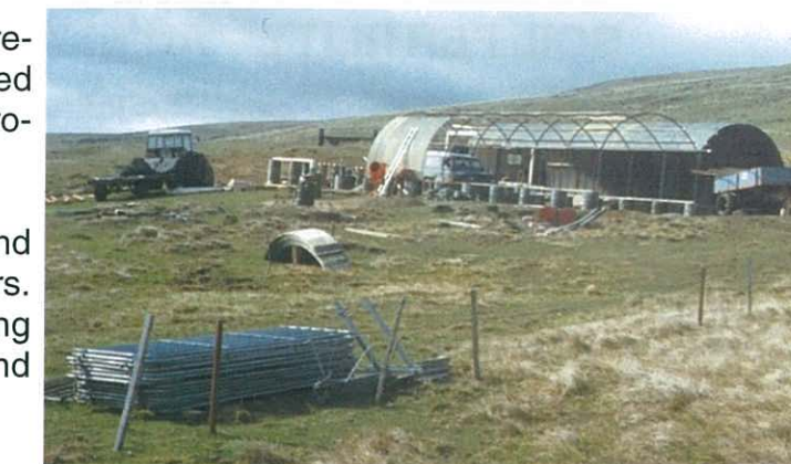
The shearing shed at Moss Side before completion
