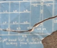
Right hand Wall of Outhouse looking from outside
