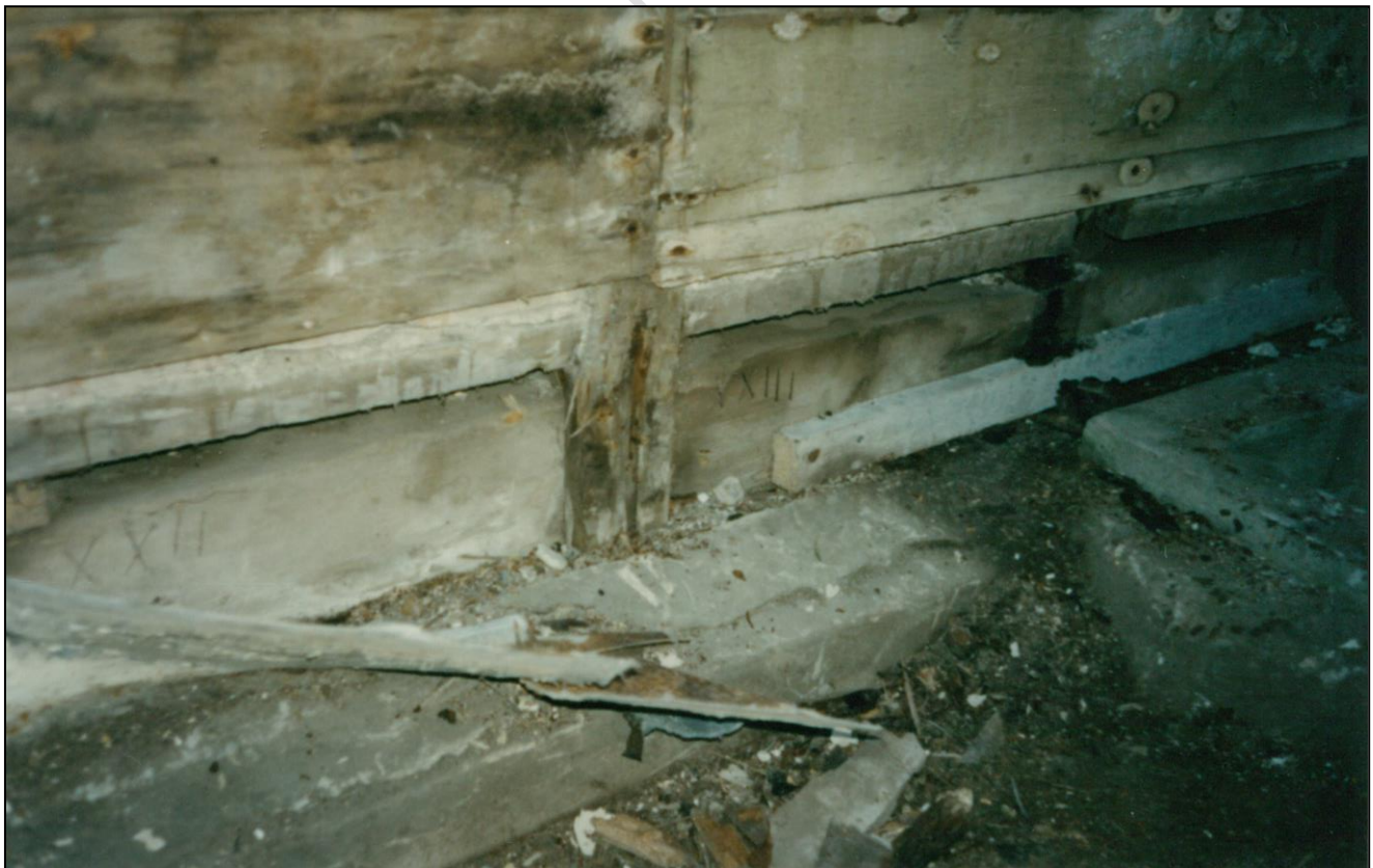
Original beams of the kit house showing the Roman numerals, etc
