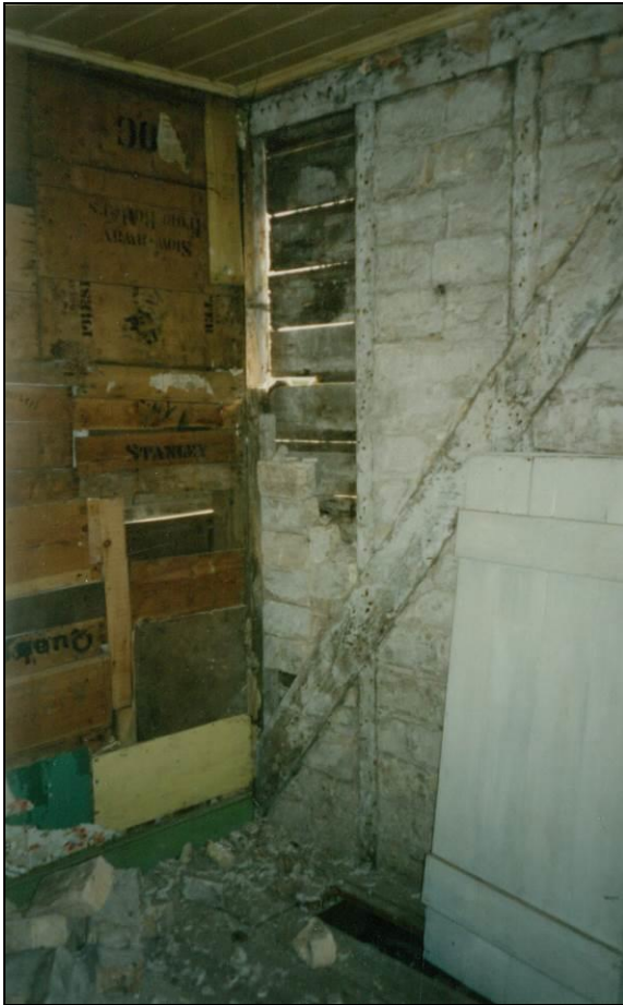
Wall coverings stripped away to expose lining material used
