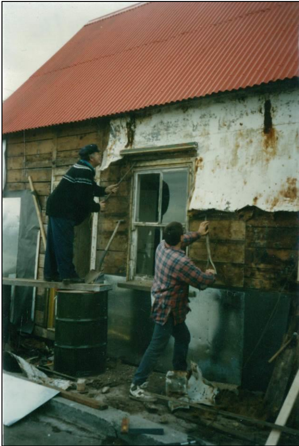
Old tin cladding being stripped off to make way for new
