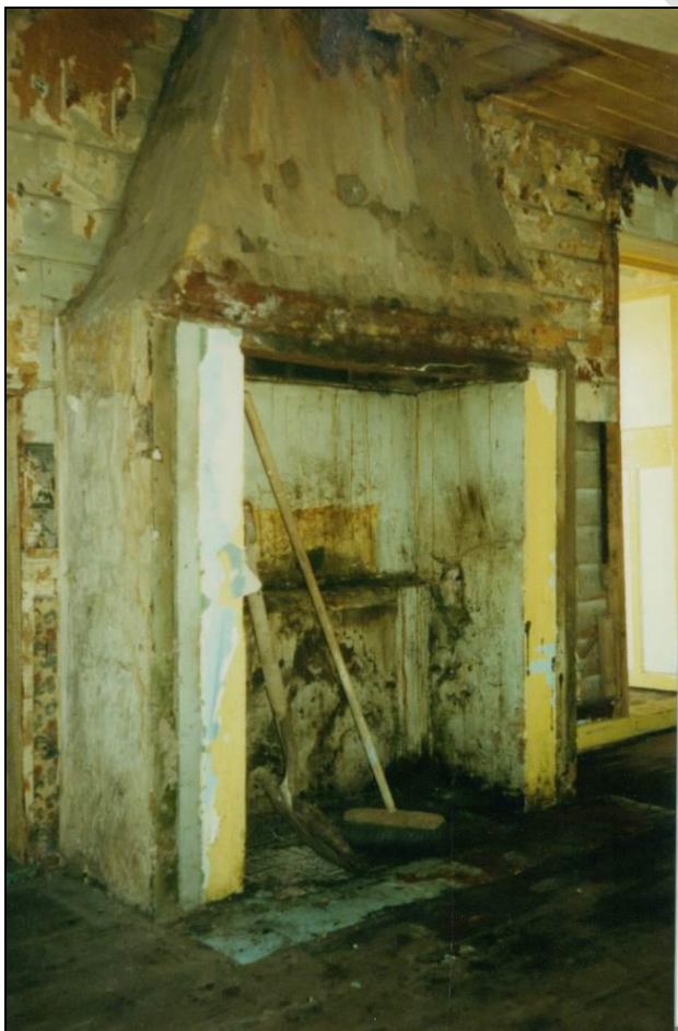
Original range being before and after removal and exposing of chimney breast
