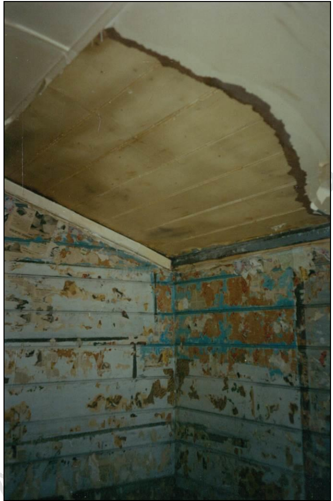
Stripping off of hardboard in other bedroom
