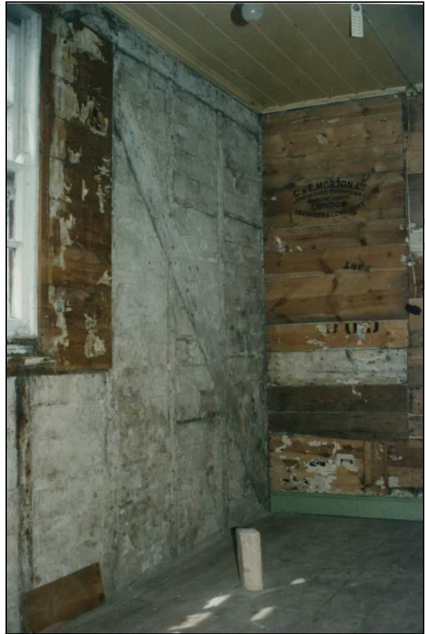
Wall coverings stripped away to expose lining material used
