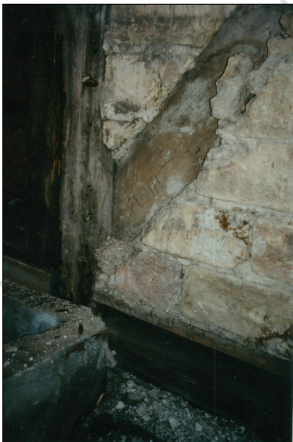
Original beams of the kit house showing the Roman numerals, etc
