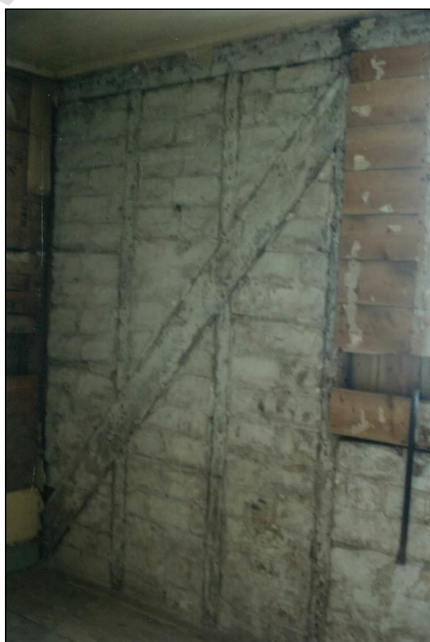
Original beams of the kit house showing the Roman numerals, etc
