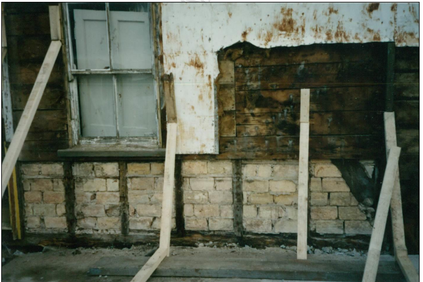
Old tin cladding being stripped off to make way for new
