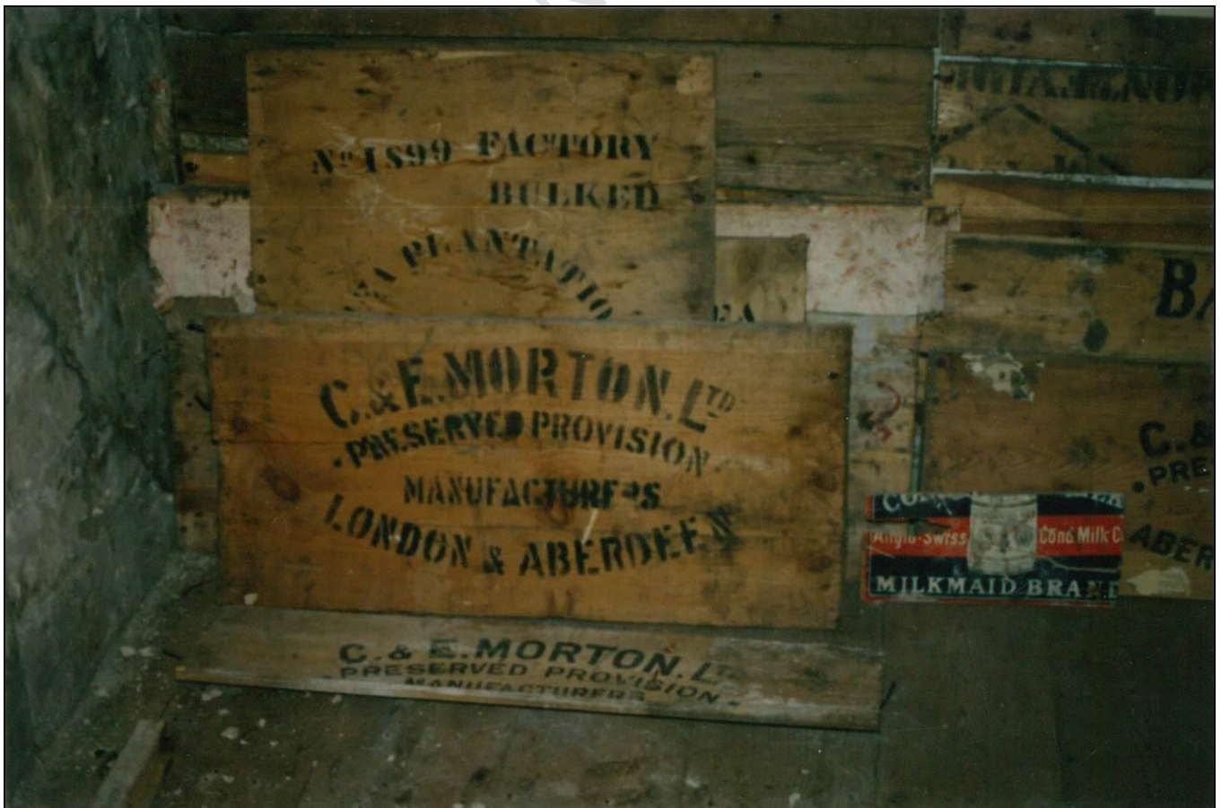
Wall coverings stripped away to expose lining material used
