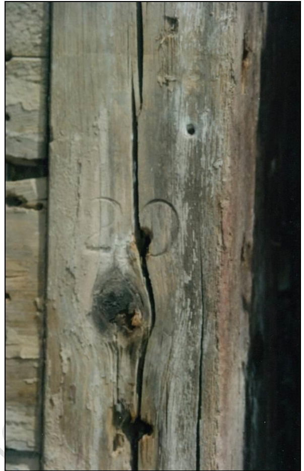
Original beams of the kit house showing the Roman numerals, etc
