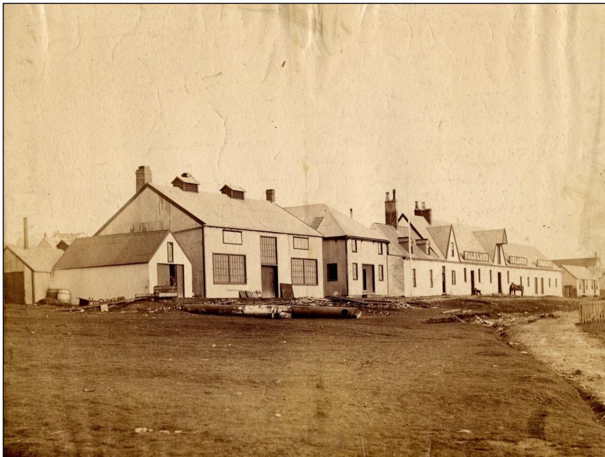
1890 – Boiler house, blacksmith's shop & store Crozier Place
