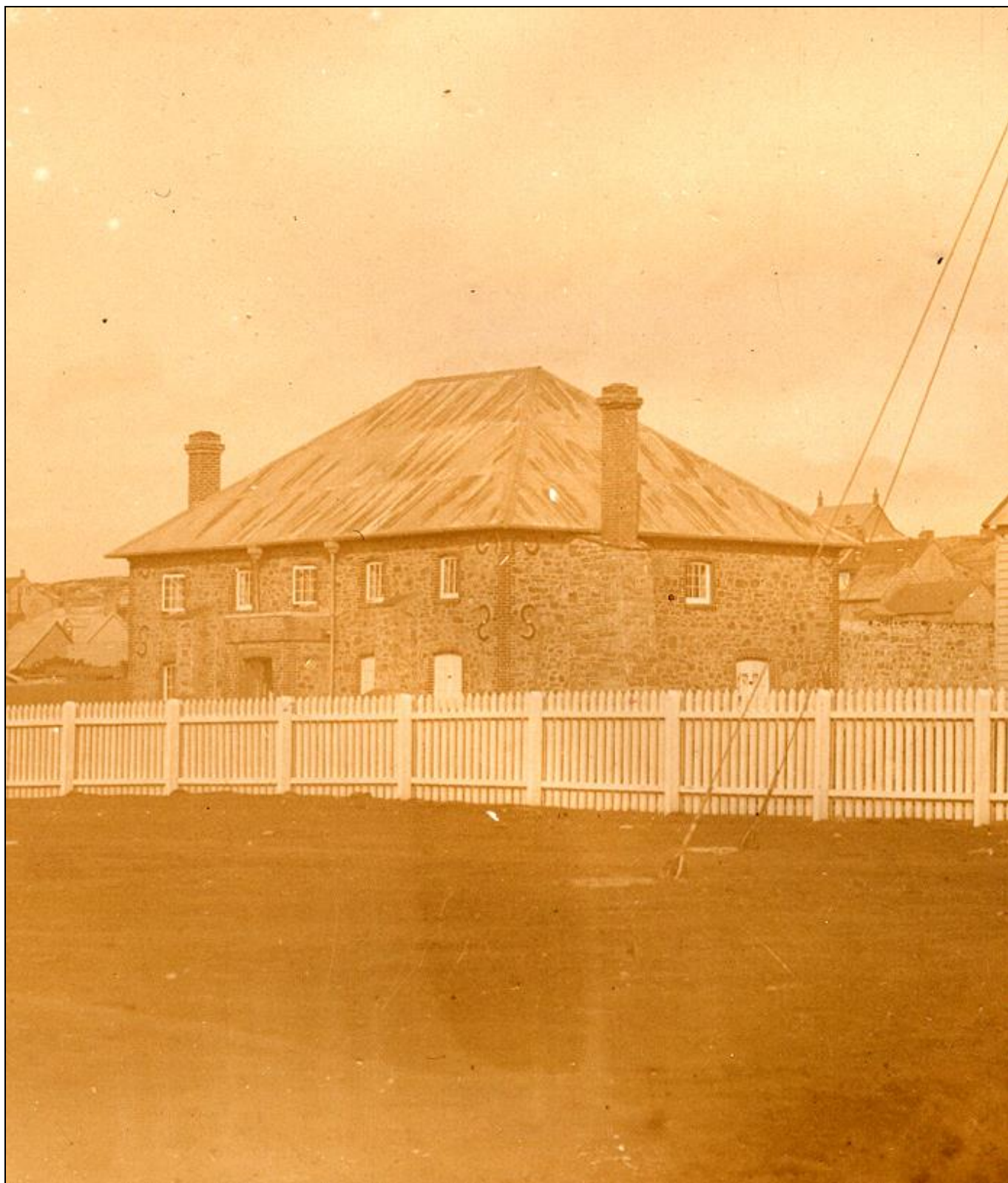
The Gaol after the fitting of the iron tye-rods – Luxton Collection
