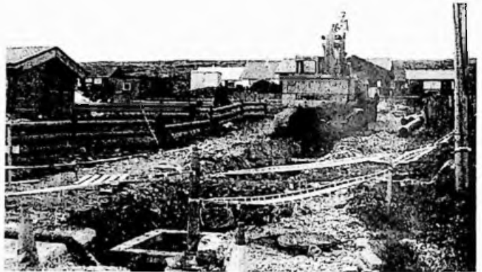
Above: A Gordon Forbes digger stands astride part of the drainage trench on Capricorn Road.
