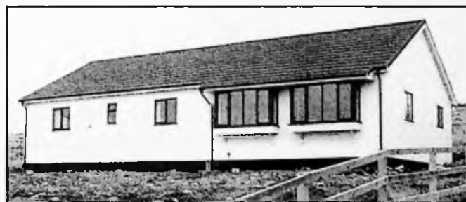
A Christian Tortsen timber frame house built by LMW Construction for Emma Edwards at East Stanley Development.
