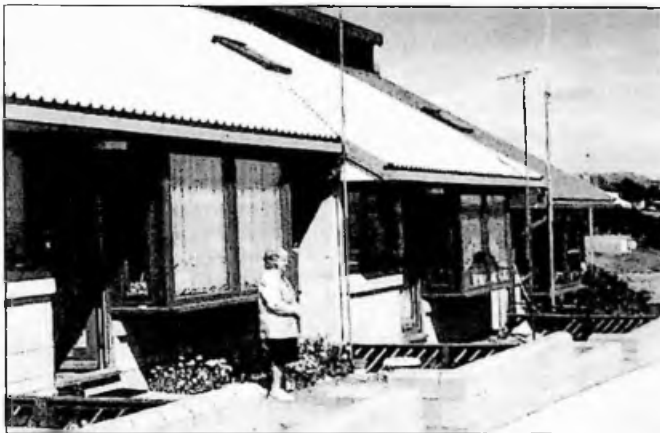
Sheltered accommodation on Thatcher Drive.
