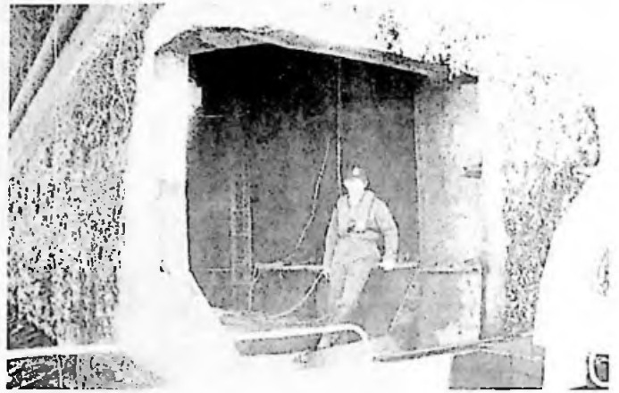
Above: Terry Bonner stands inside the barge following the removal of the bent and twisted metal caused by the collision with the Siera Gredos
