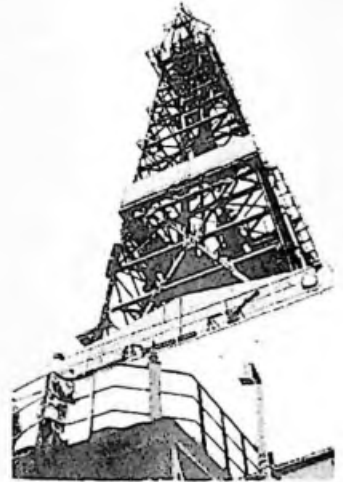
On board oil rig Borgny Dolphin in the North Falklands basin in 1998.
