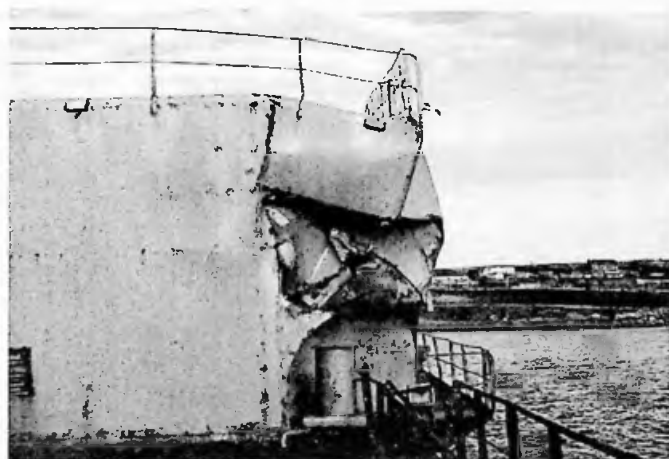
Above: The damaged barge at FIPASS
