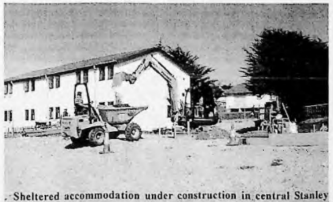
Sheltered accommodation under construction in central Stanley
