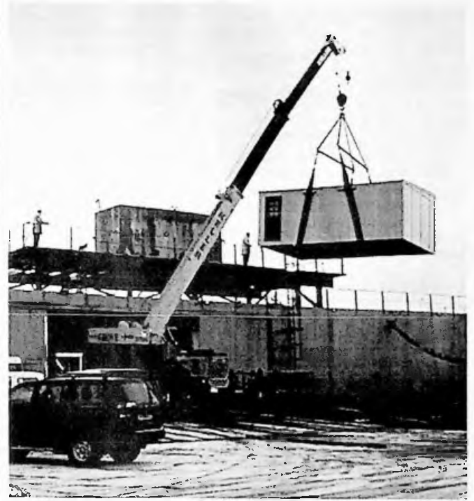
The hatchery is lifted into place on FIPASS
