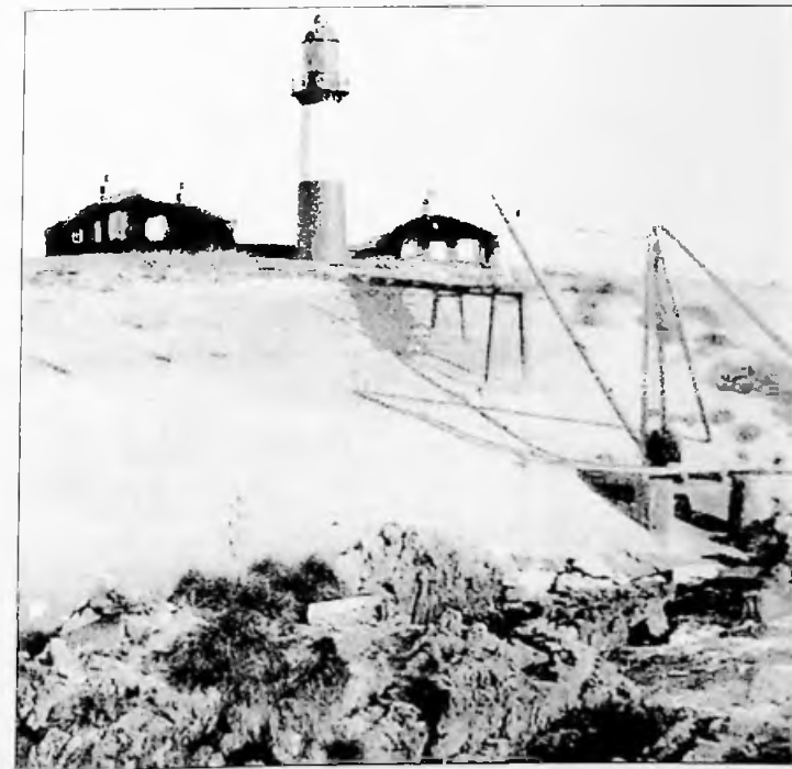
Above: The landing stage and crane pictured to the right was constructed from steel salvaged from the jetty which was destroyed in 1906.
