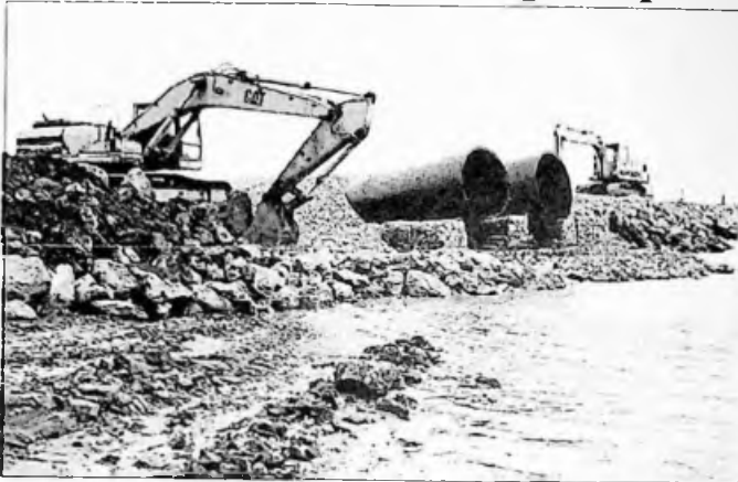
Above: Work on the Corral Creek culverts underway on Tuesday
