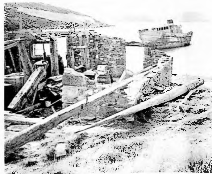
The results of the September 2000 hurricane force winds. Note the ship's mast which had been a horizontal support for the roof trusses. This was snapped into four pieces, with the main section of the roof taken 100 metres up the valley.
