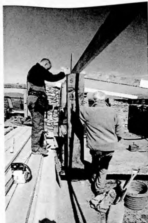
The oak ship's timbers being positioned on their original footings. These support the main roof section and form an important feature in the building.
