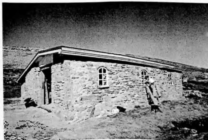
The building with completed roof. The "photographer" and volunteer painter working on the specially made arch windows. A view to the SW. November 2005
