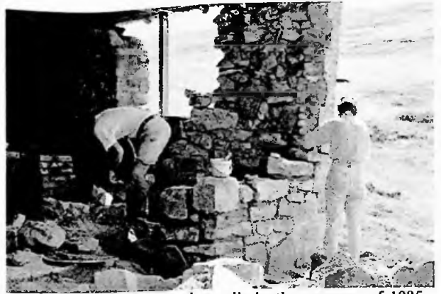
Main reconstruction on the walls in the summer of 1995 - 1996. The building's roof at this stage was believed to be some 60 years old and survived without a single holding down strap into the stone walls. A second interior wall was constructed to support such sections as shown here.
