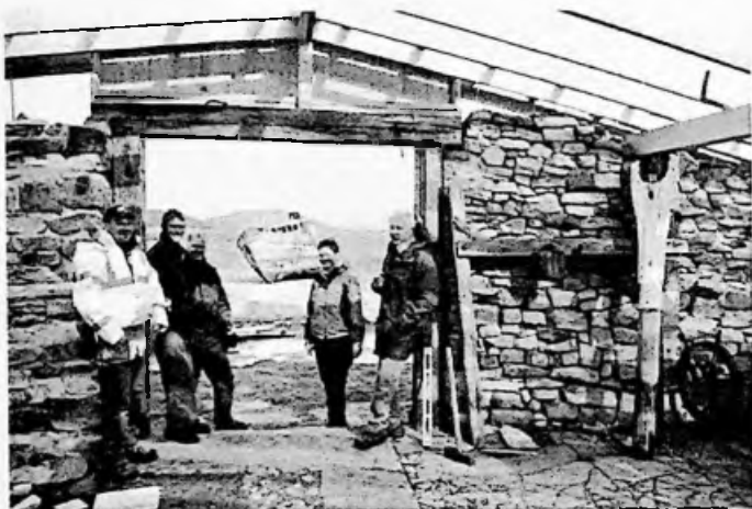
Ian Stewart Construction and his volunteers. October 2005 and the new roof trusses are complete. A view from the interior looking out over the Protector beach and SE.
