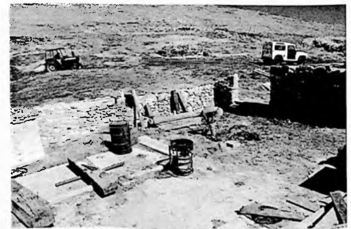
Clearing the site early October 2005 in preparation for the second attempt at restoration
