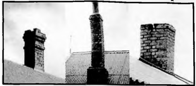
Examples of the poor condition of some remaining brick chimneys
