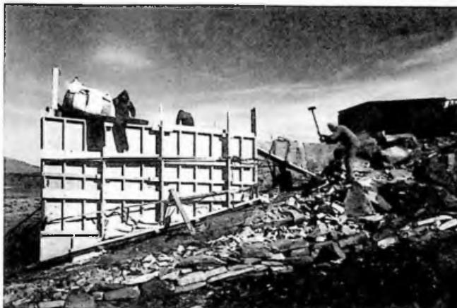
The Construction Site: Wooden shuttering was put in place around the existing jetty wall to hold the new concrete.
