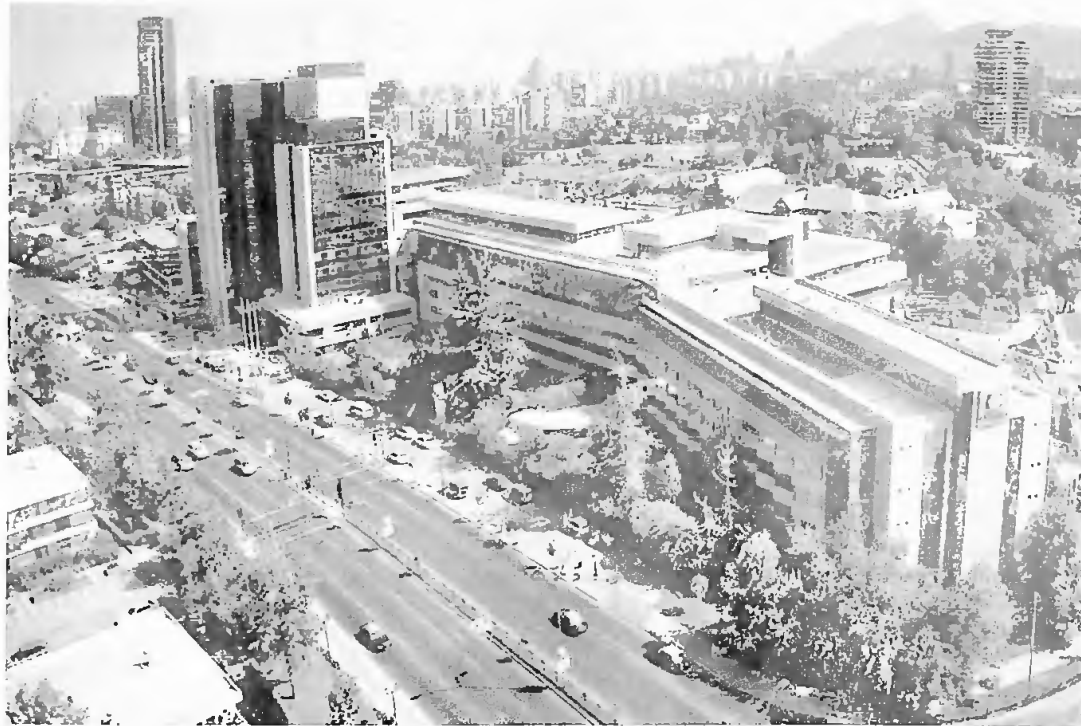
Above: An aerial view of Clinica Alemana - the towering Marriott Hotel can be seen in the background.
