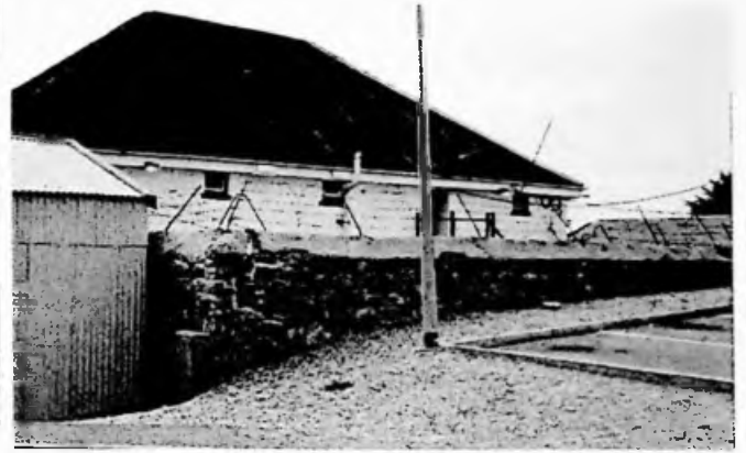
View to the rear of the Stanley Police Station and Prison showing part of the prison yard.
