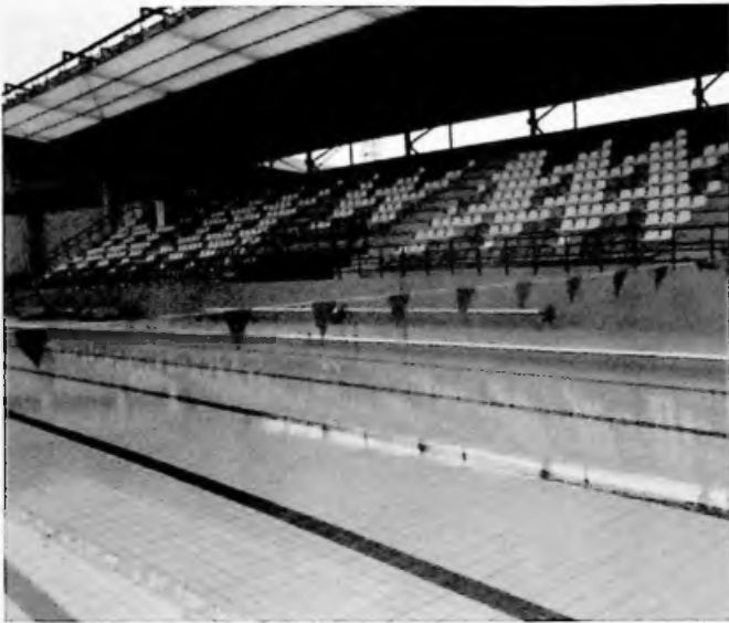
Above: The Nigeria pool
