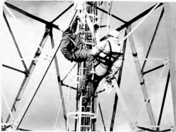
ABOVE: Members of Cable and Wireless's transmission and provisioning departments have been put through their paces - high in the air.
