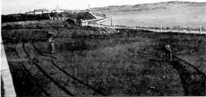
Howell Evans supervises the laying of the lower garden, 1945.
