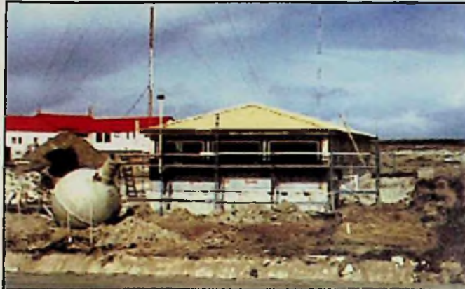
Above: The fuel station under construction on the Stanley By-Pass Road
