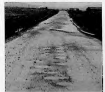
Above: The Moody Brook Road
