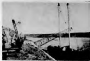
Above: An improvised crane: One of many pictures depicting the construction.
