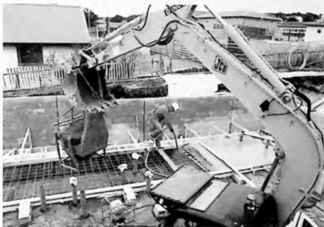
Above: The concrete pour gets underway on the new prison block - tunnelling out will be a daunting task for any 'great escaper'.
