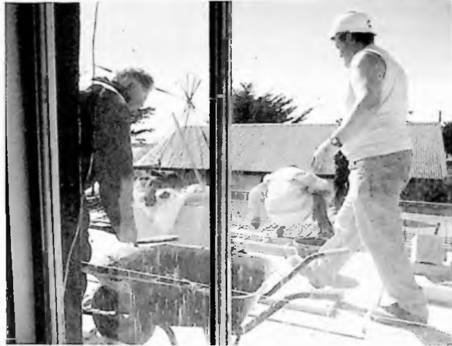
Above: At window level Bricky Alan Ross and Peter Villegas keep up a steady pace with the block work.
