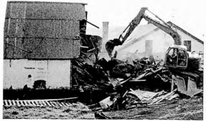
The demolition of FIC's Basics shop on Dean Street
