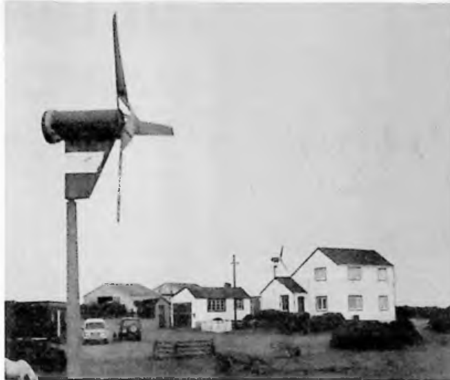
Wind turbines at Hill Cove supplying power to residents
