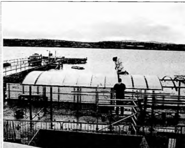
Morrison staff work on a new shelter at the public jetty
