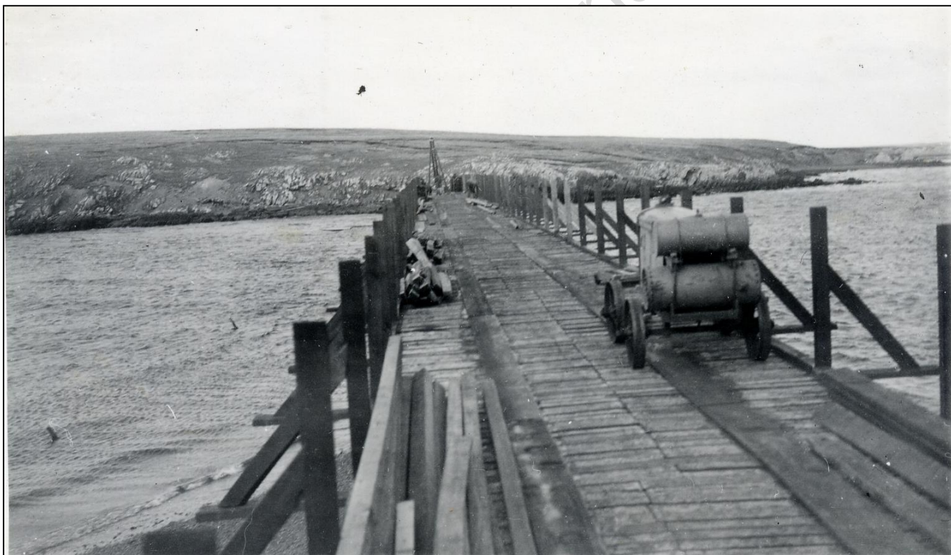
Paterson's Point Bridge under construction – FIC Collection, JCNA
