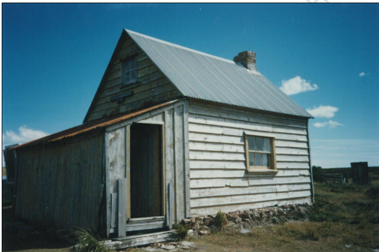
The Lochhead Shanty which was originally built from the wreck of the Carlton at Cow Bay and later dismantled and rafted up Loch Head Pond and re-erected as a boundary rider's house by George Patterson SMITH – photo JCNA
