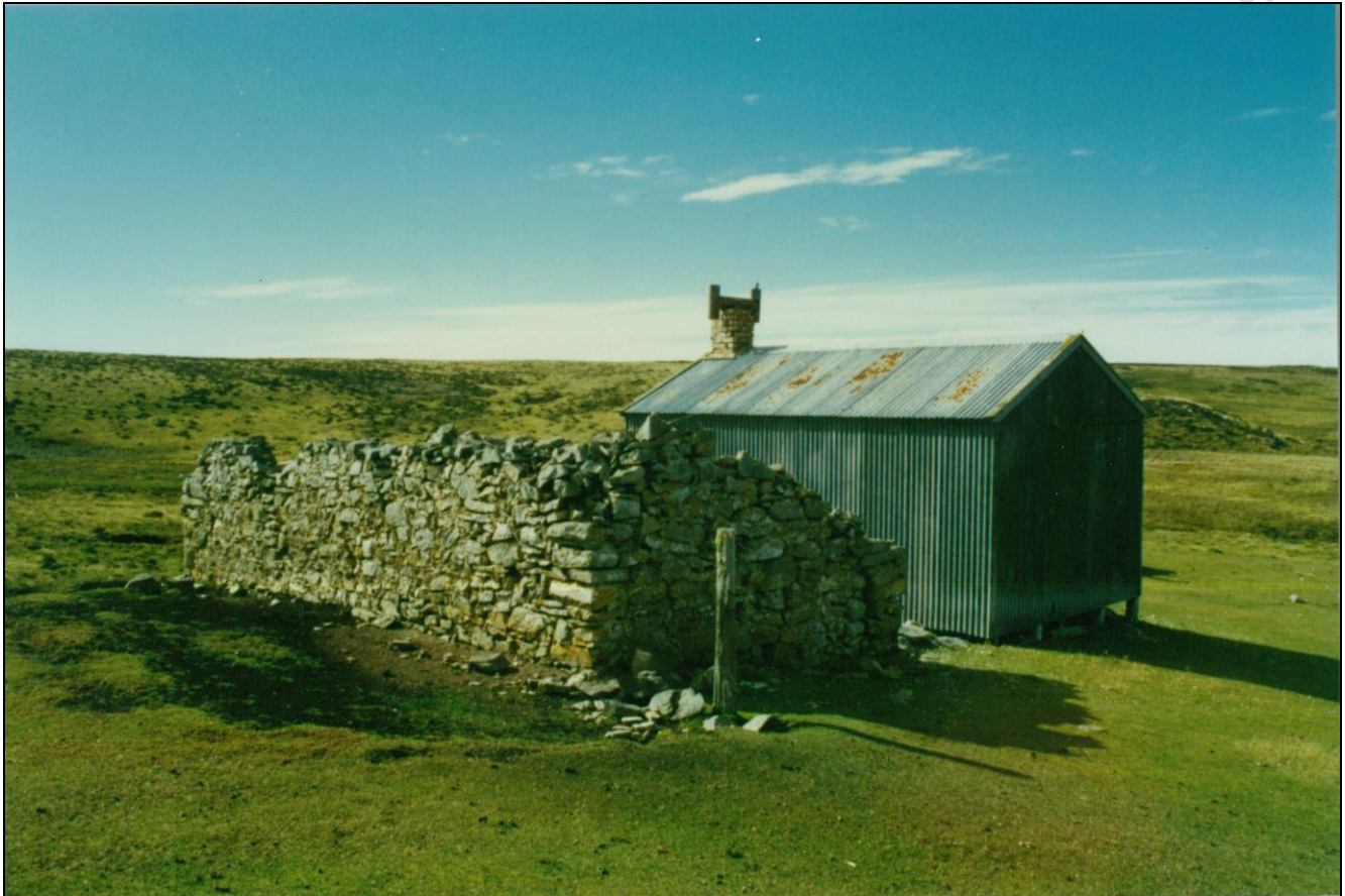
Remains of stone house at Diamond Cove with the Diamond Cove Shanty in front, 1997 – photo Don Aldiss Collection, JCNA
