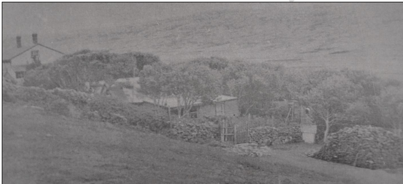
L-R The 'new house' and the 'old farmhouse' from the south east
