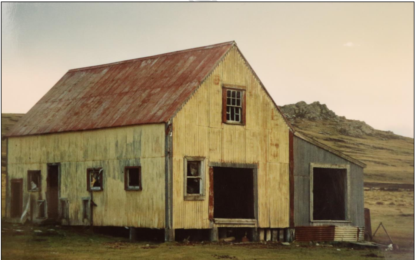
The wool shed - note the same wooden piles as the old farmhouse - 1992
