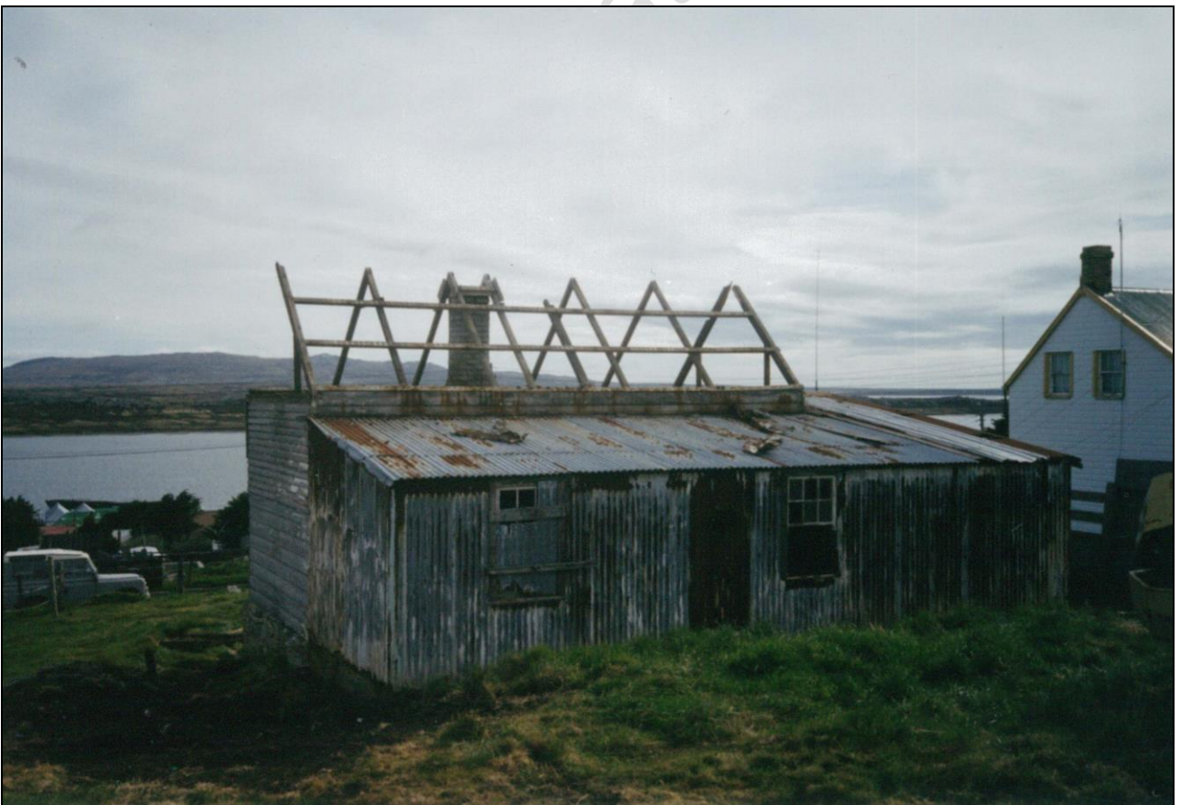
South side showing lean-to
