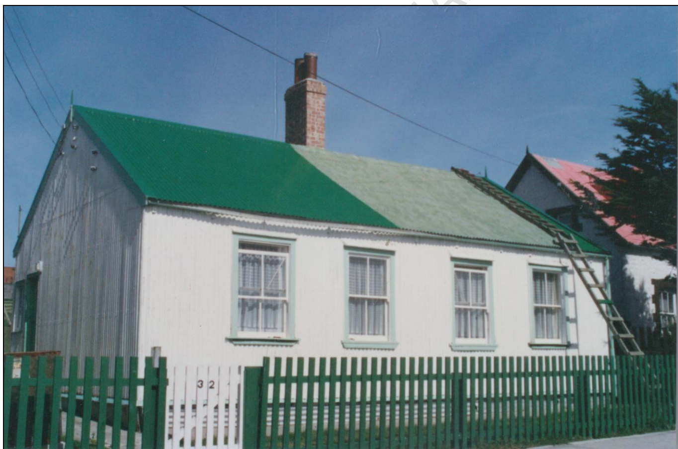
32 Davis Street from the north-east 2019 - JCNA
