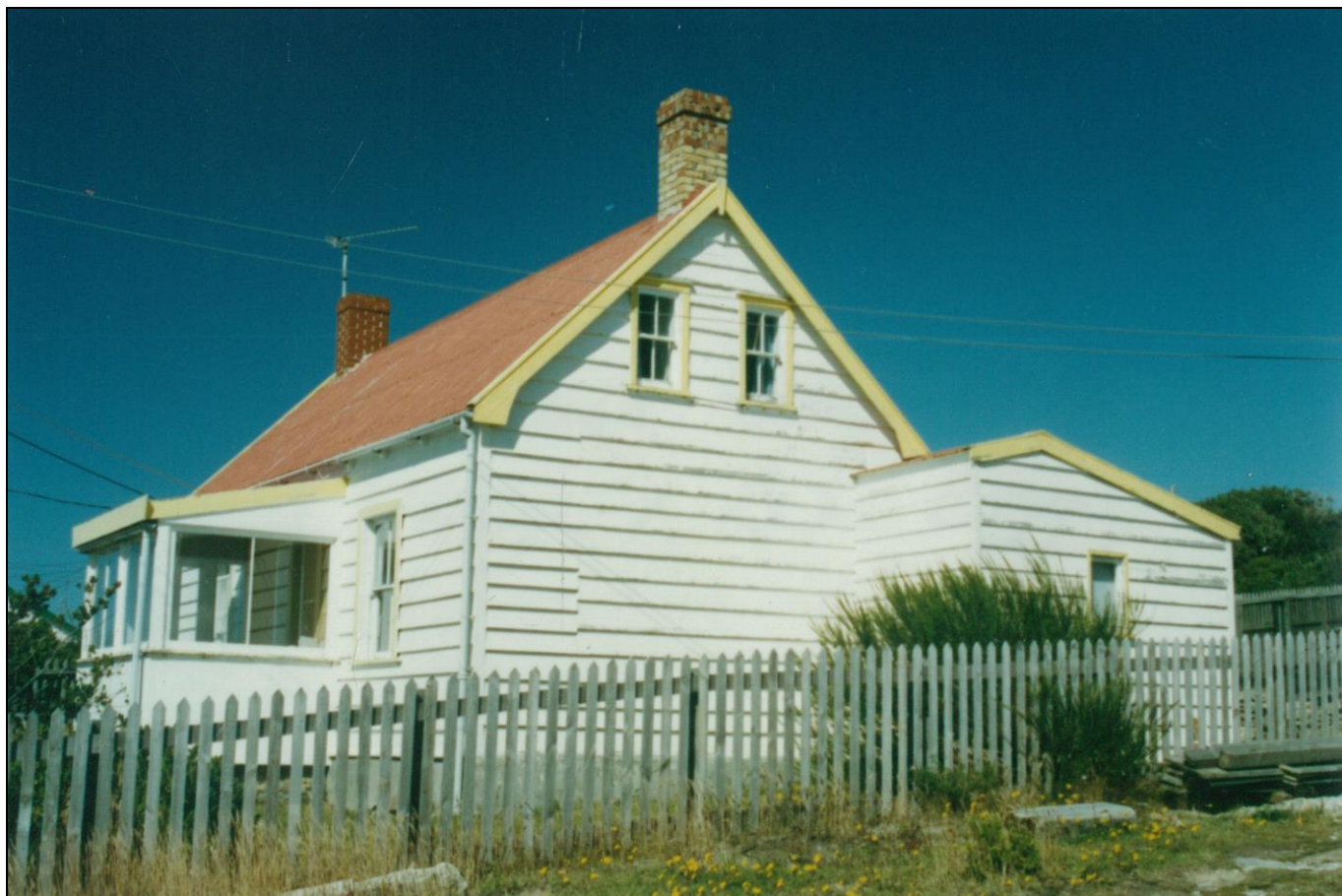
8 Ross Road East from the north west, 1992 - JCNA
