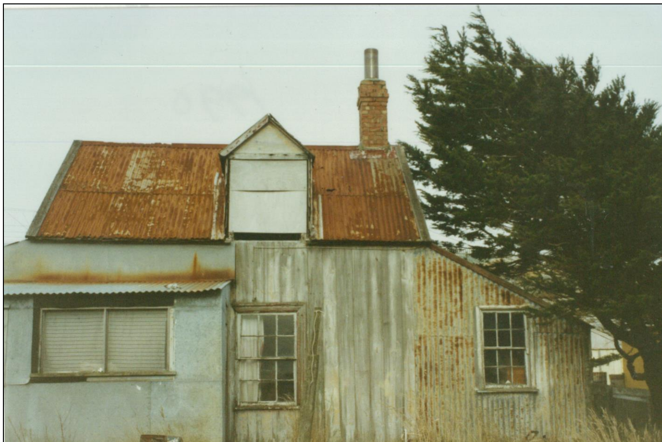
18 James Street from the north, 1990 - photograph JCNA
