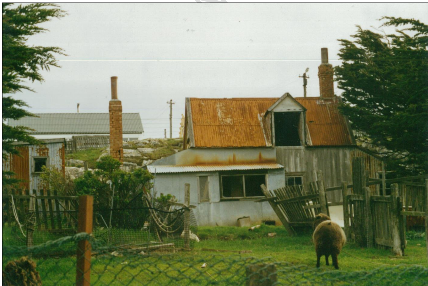
18 James Street from the north - photograph JCNA
