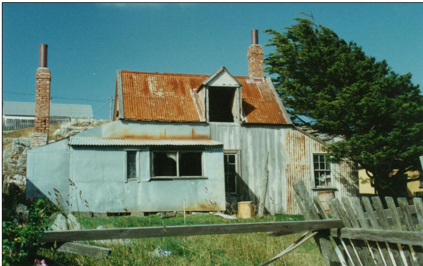
18 James Street from the north, 1993 - photograph JCNA
