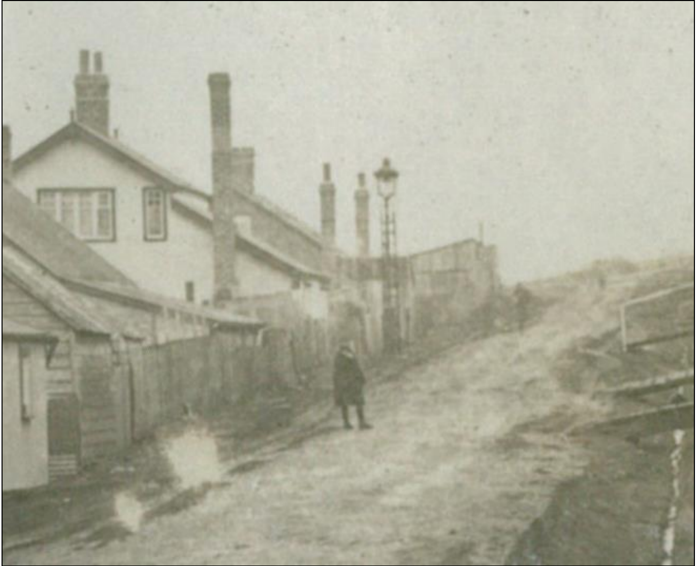
9 James Street from the south west (first house, partially obscured by No 7), 15 June 1925 - photograph JCNA
