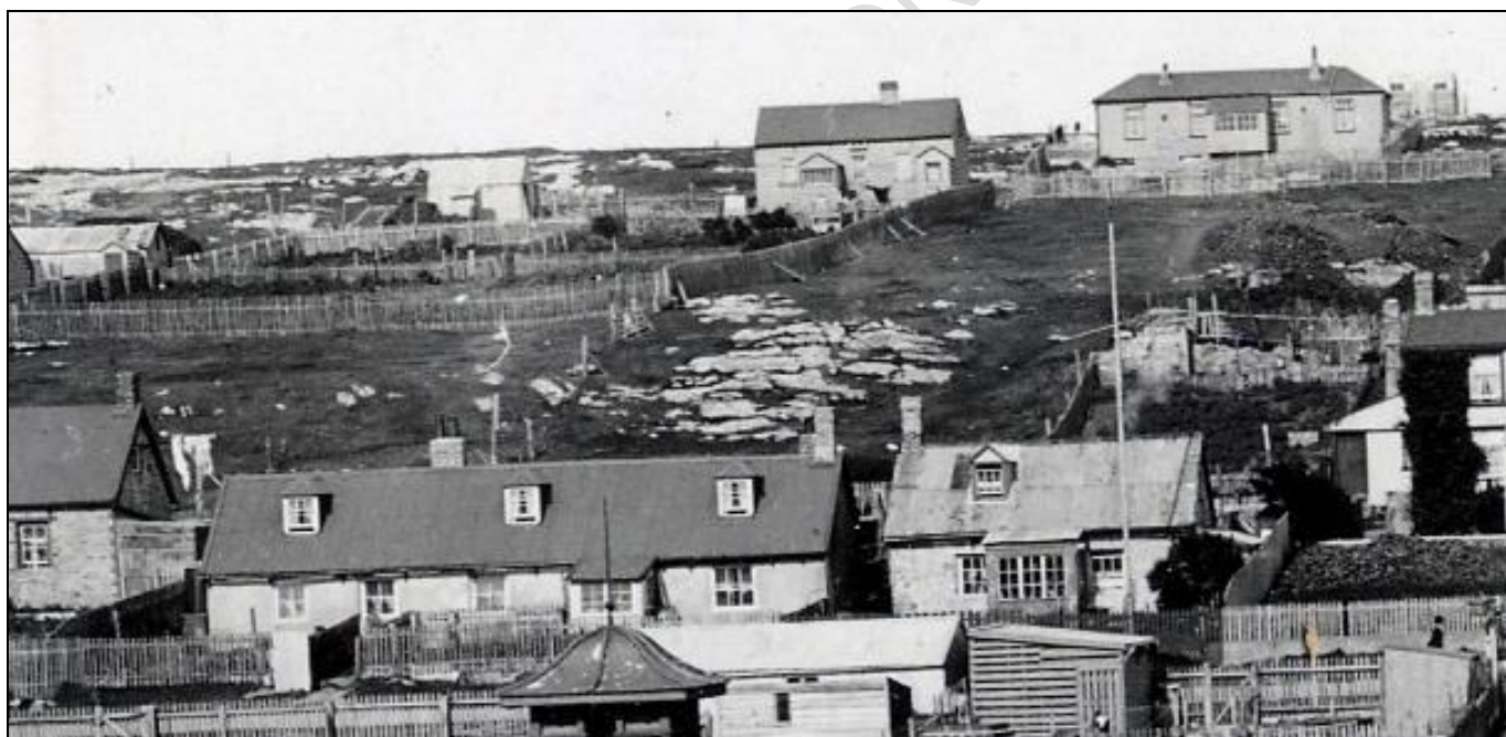
Front centre L-R: 33 Fitzroy Road and 31 Fitzroy Road in 1927 - FIC Collection, JCNA
