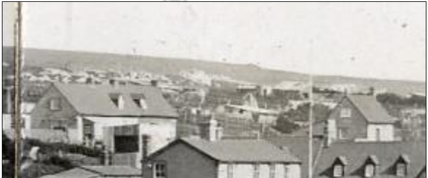
Early 1927 – Left-hand half of semi-detached house back-left is on PCA 27
