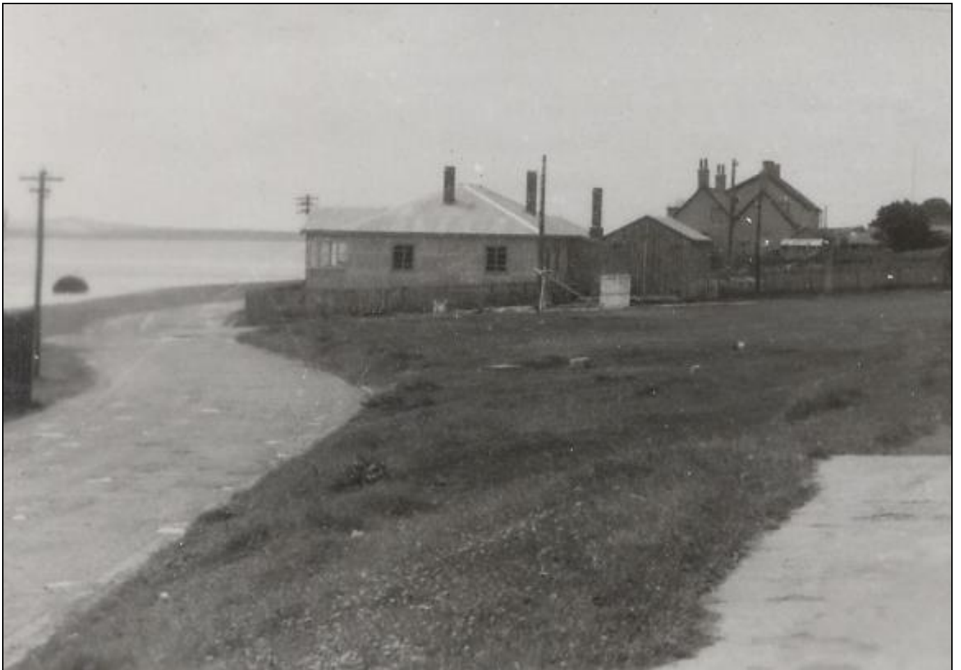
Post January 1946 showing a house built on the corner of the site - FIC Collection, JCNA
