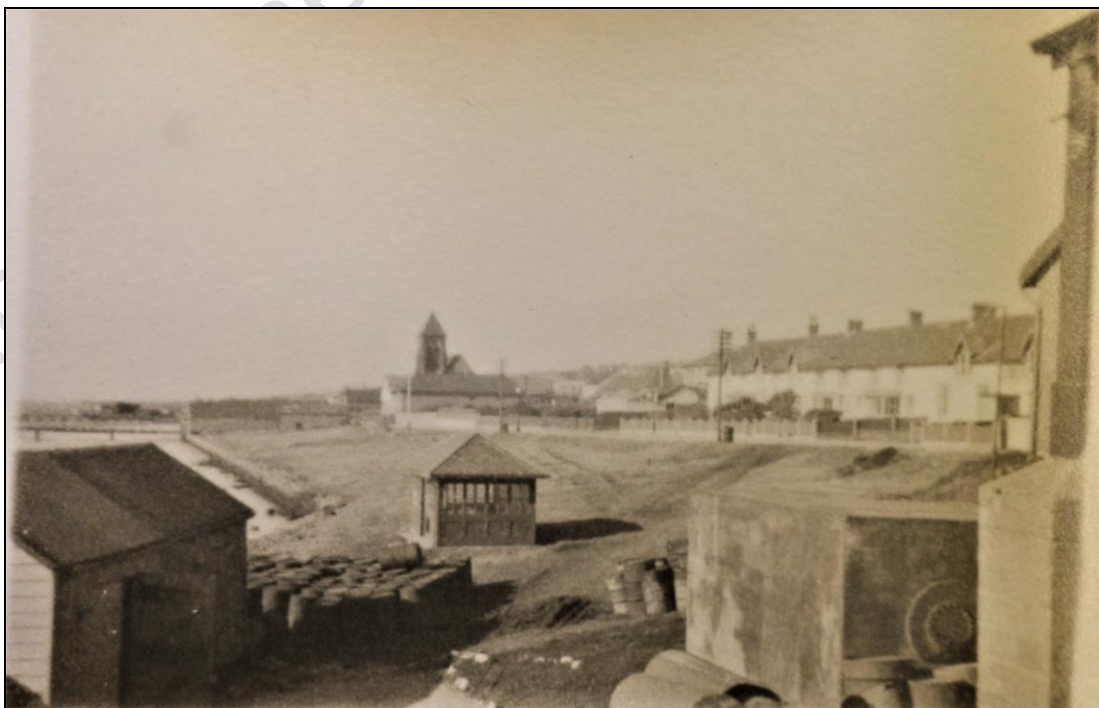
Foundation building, new Town Hall looking south east – Tony Carey Collection, JCNA
