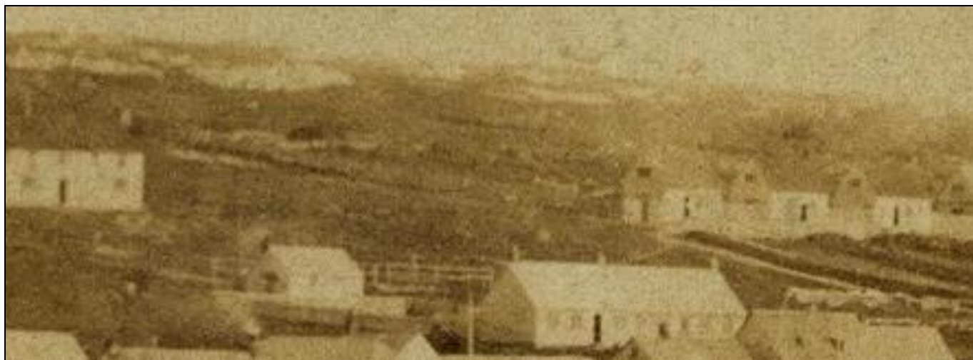
1863 - Large house front centre
