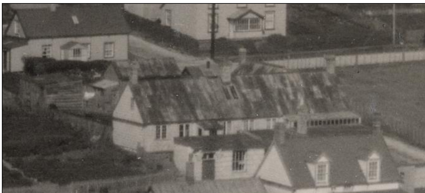
1936 - Large house in centre with store partially obscured in front - FIC Collection, JCNA
