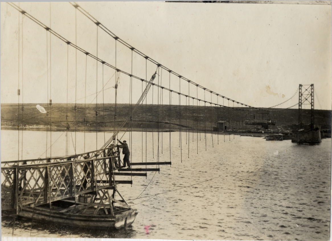
ERECTING GIRDERS
