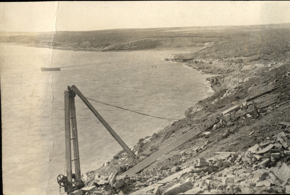
Excavations for Anchor Hole D. side.
