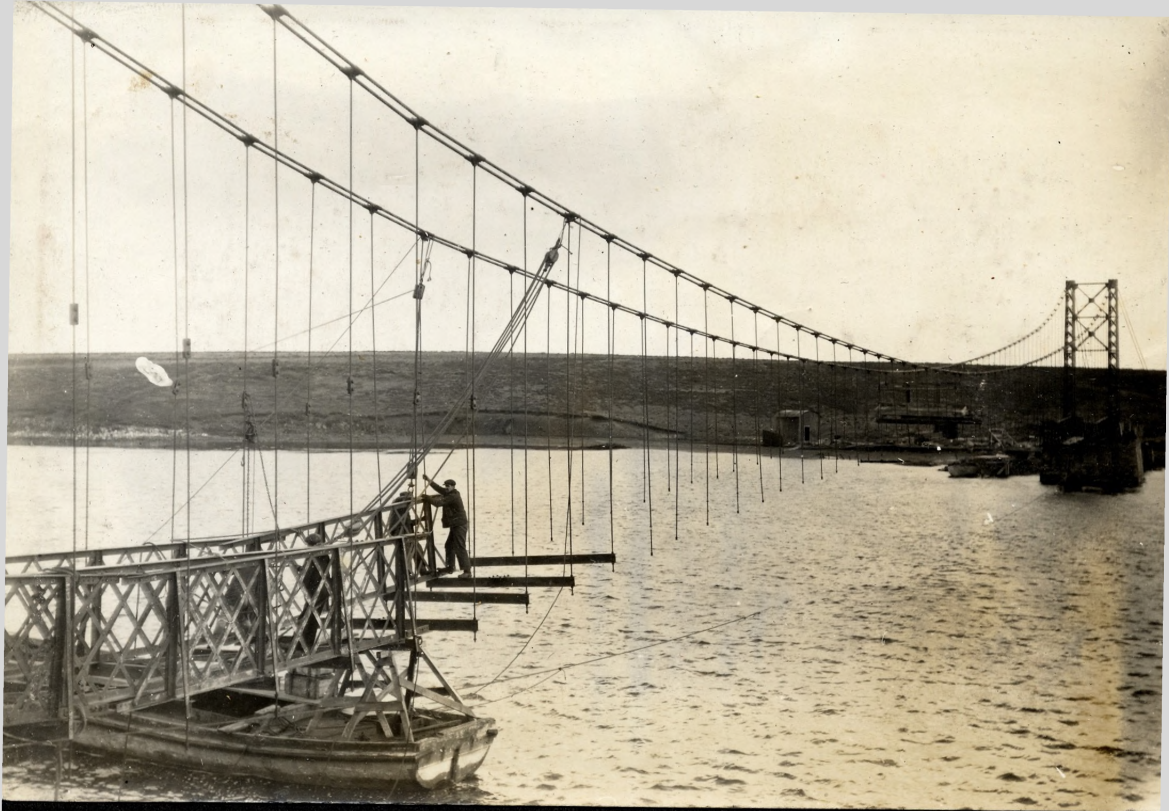
Erecting Girders.
