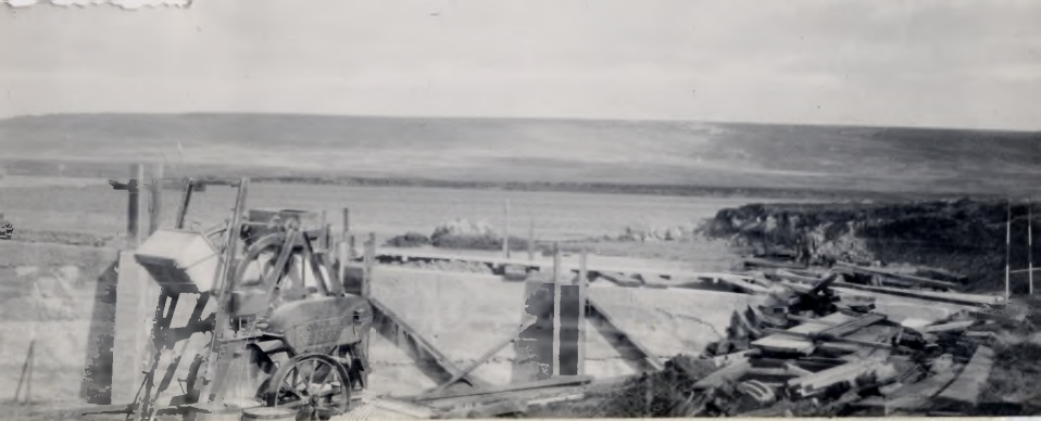
Building Paterson's Point Bridge.
