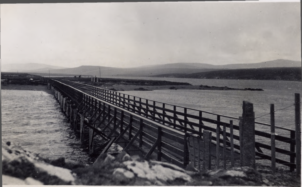
THE BRIDGE COMPLETED
