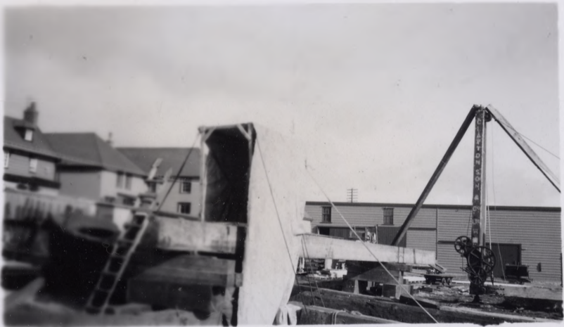
SAWING BEARERS FOR FITZROY BRIDGE
