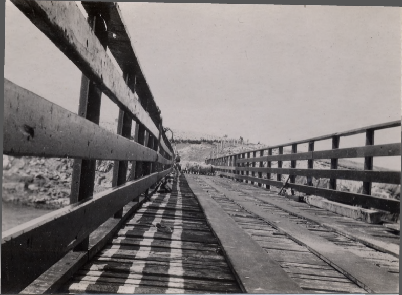
PATTERSONS POINT BRIDGE, FITZROY
