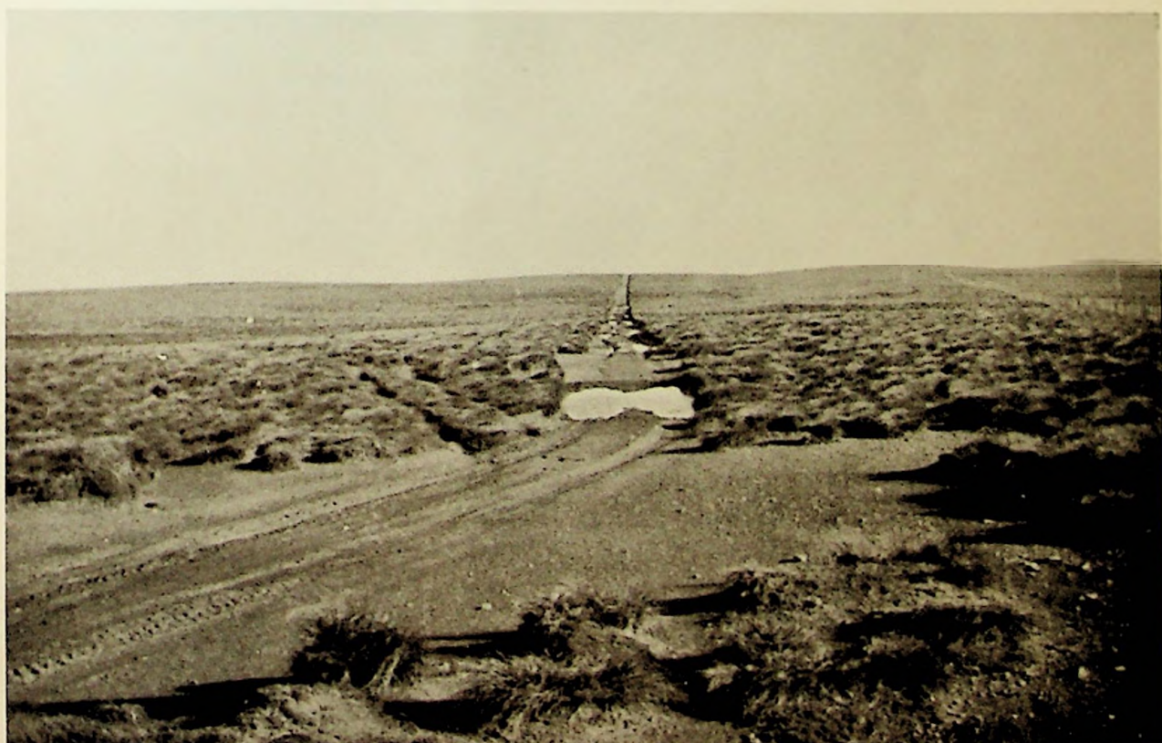
PLATE II. Poor drainage and lack of maintenance on Fitzroy-Darwin track.
