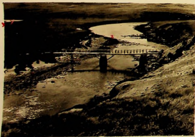
Nos 4 & 5. Existing wooden bridge approximately 1\frac{1}{2} miles above Site "B". Shows the erosion which is taking place on left bank and the spit of ground which it is reported occasionally floods during Winter. Site proposed for bridge marked "X" on No 4. photograph.
