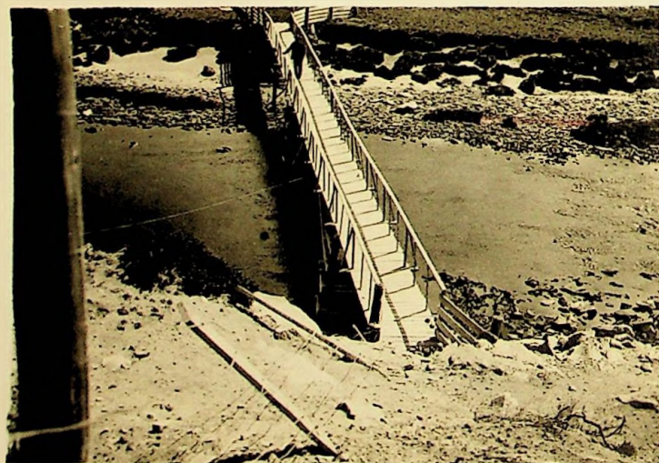
Nos 4 & 5. Existing wooden bridge approximately 1\frac{1}{2} miles above Site "B". Shows the erosion which is taking place on left bank and the spit of ground which it is reported occasionally floods during Winter. Site proposed for bridge marked "X" on No 4. photograph.
