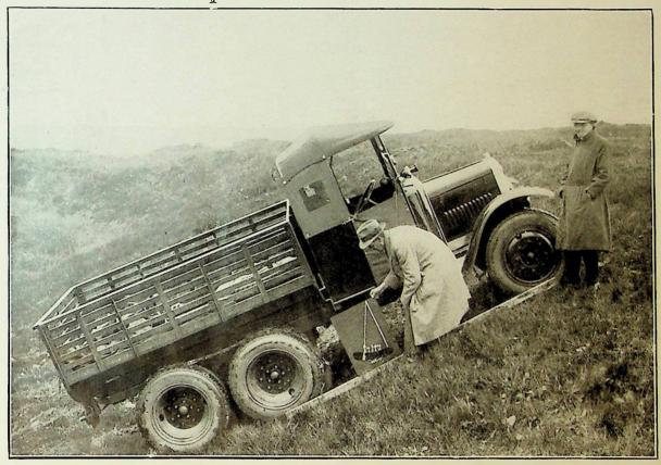
In its normal form, and without any additions, the Morris-Commercial Six-Wheeled Vehicle will negotiate almost any conditions that are likely to be encountered. For use in cases where deepsided and slippery ditches or hillocks have to be overcome, however, chain tracks are provided which fit round the four rear driving wheels. The task of applying these chains is extremely simple—quite as simple as fitting of non-skid chains on to an ordinary vehicle.
