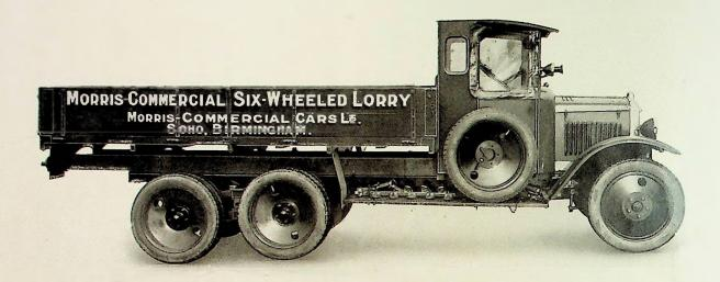
The above illustration shows the 2-ton model with a 12 ft. lorry body mounted. This body has a width of 5 ft. 6 in. and the sides are 18 in. high. As shown below, the sides and tailboard are hinged, and if desired can be removed, thus enabling the machine to be used as a flat platform carrier. The price of this vehicle complete (without side-curtains) is £505.
