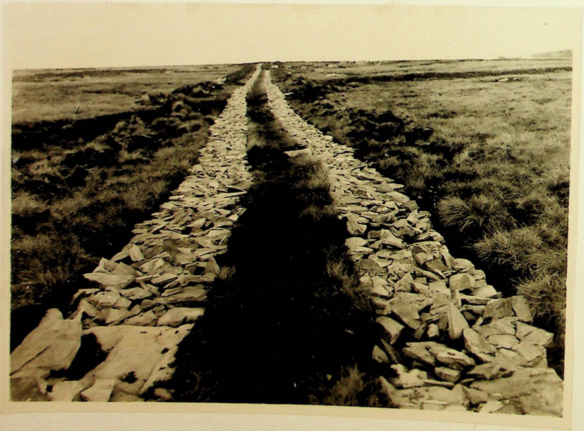
A length of track through a grassy peat bog filled with rock to form mattress. The rock has yet to be hand knapped and covered with peat loam.
