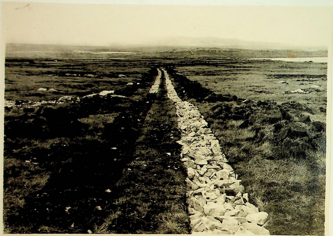
Track passing through a peat bog with outcrop of rock. The portion of the track on the left has been hand knapped and covered with peat loam.
