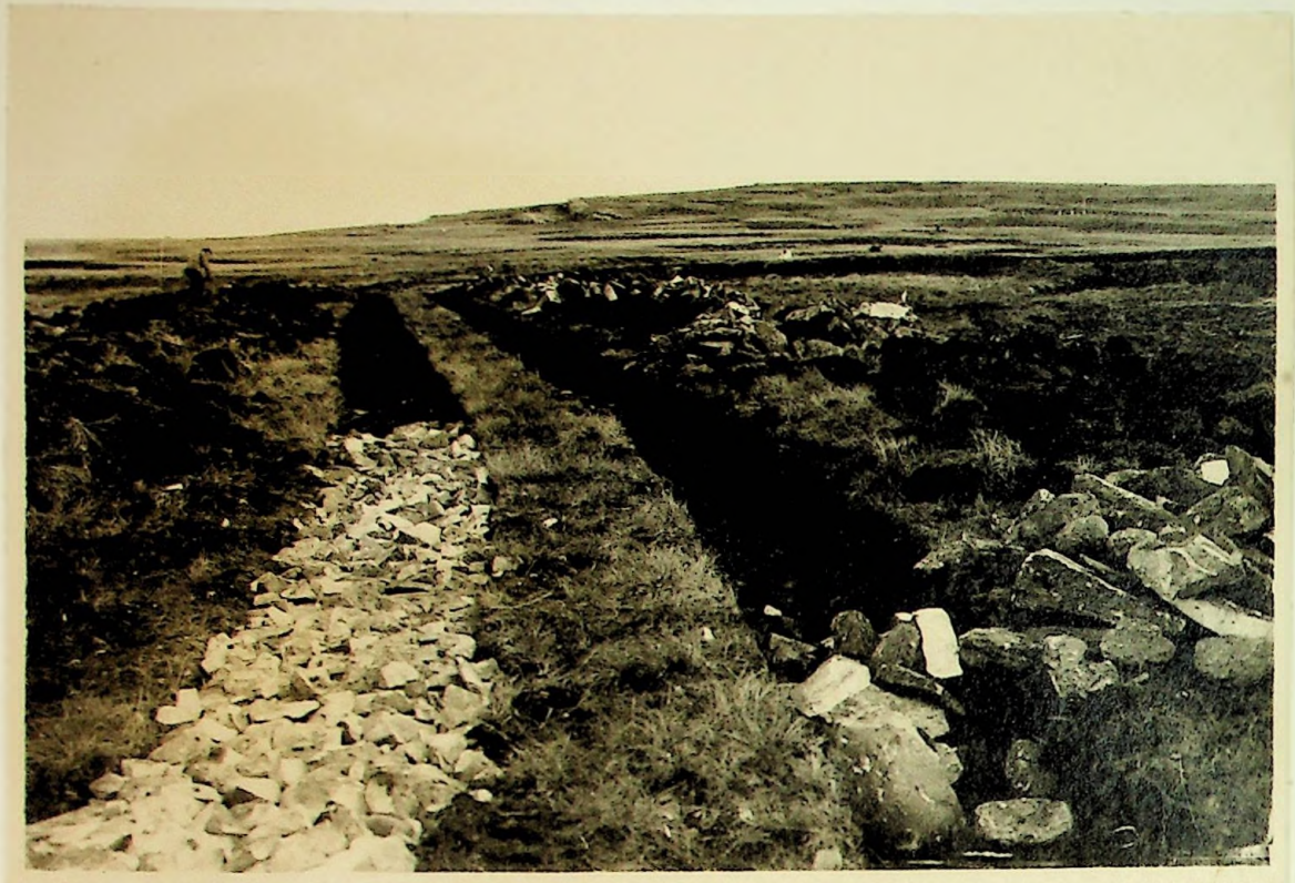
Background shows trenches cut 2' 6" wide and 1' 6" deep, and in course of being filled with rock to form mattress for track in foreground.
