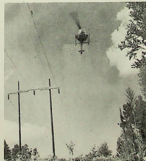
Keeping the routes of power lines free of weeds by use of "viscous water" sprays
