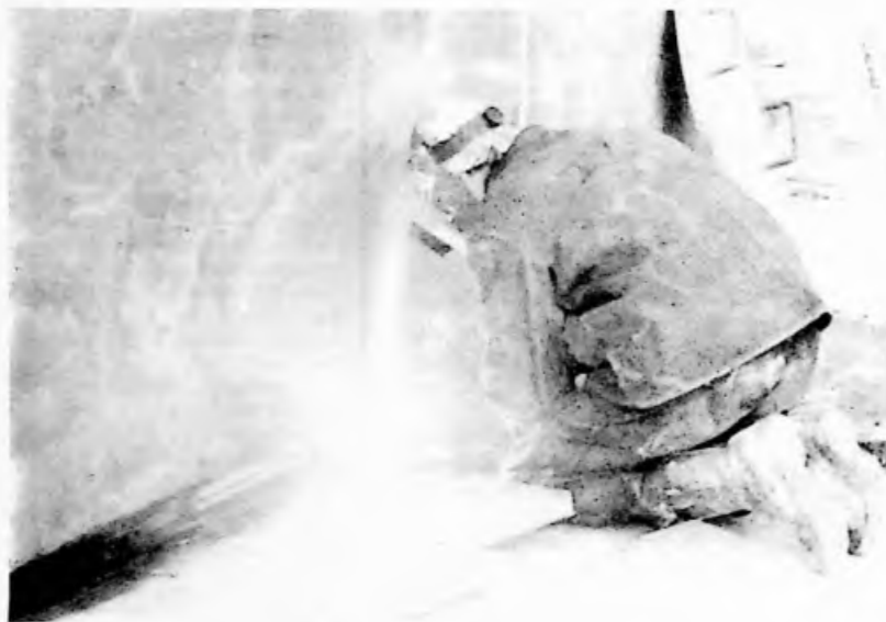
Welding one of the 2.5 million litre tanks
