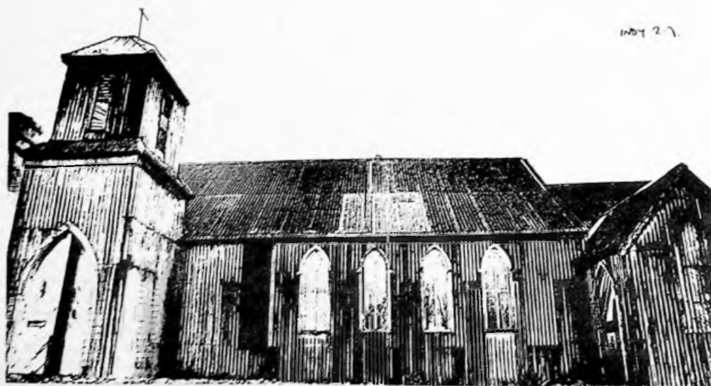
The 'rusting tin church' that is, in fact, an exceptionally elaborate example of a Victorian tabernacle
