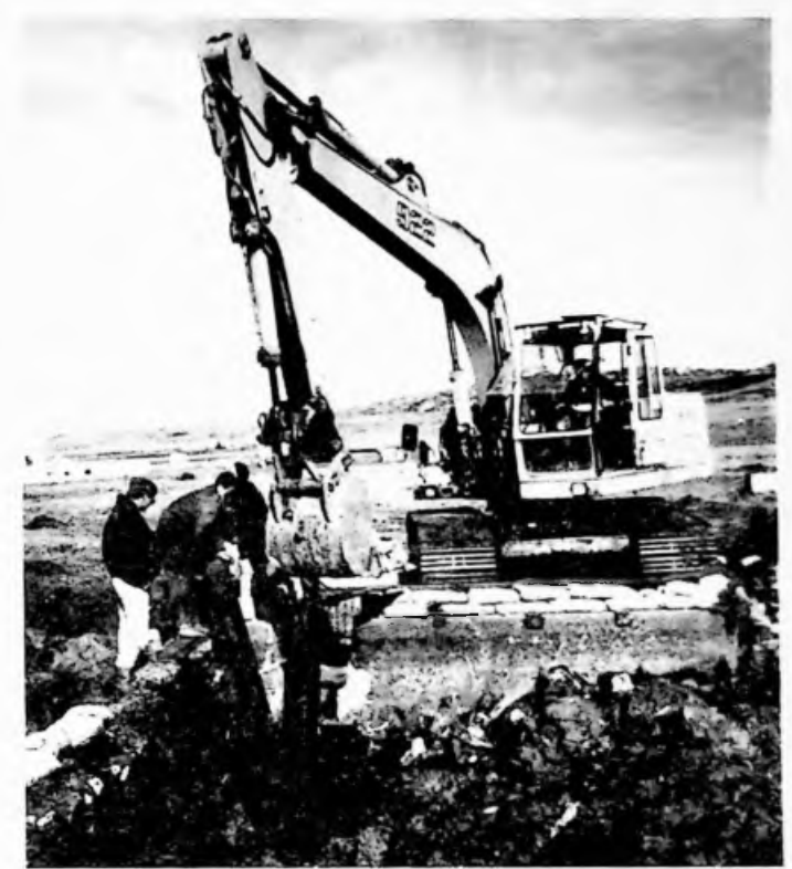
Neil McKay's excavator driving in piles probably, in the estimation of DPW, Mr. Brian Jarvis-Hill, for another fifty years.
