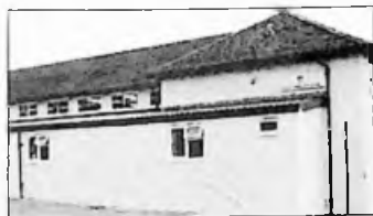
Infant/Junior School toilet block finished after eleven months
