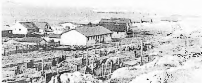
The Morrison Construction Group will be looking at Phase 5a of East Stanley Infrastructure. Above East Stanley Development.
