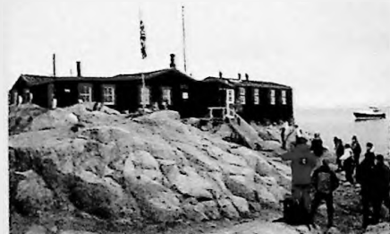
Bransfield House at Port Lockroy
