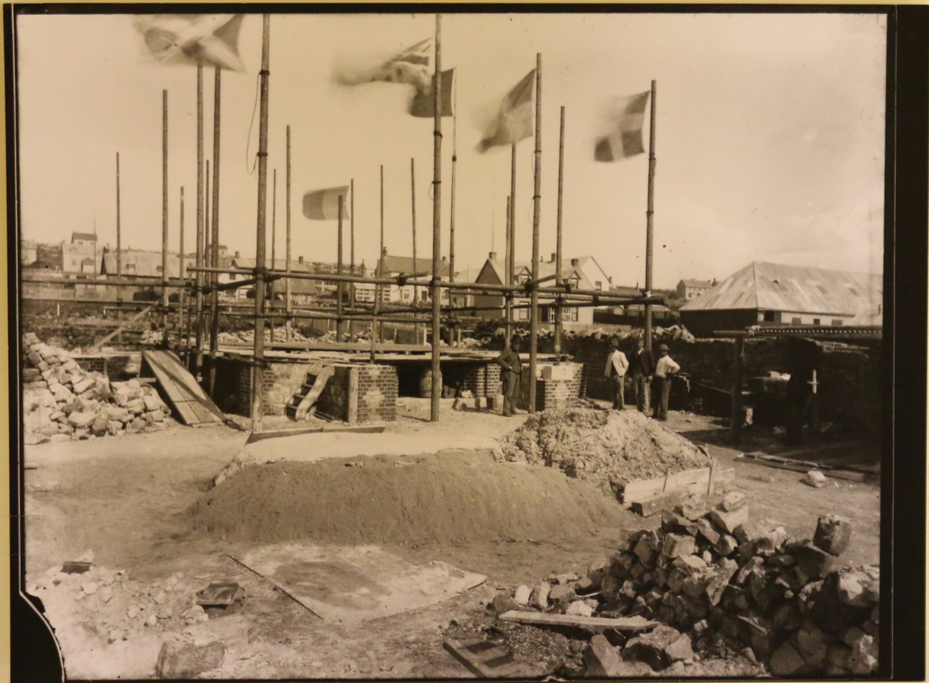
Foundations of Christ Church Cathedral c 1890
