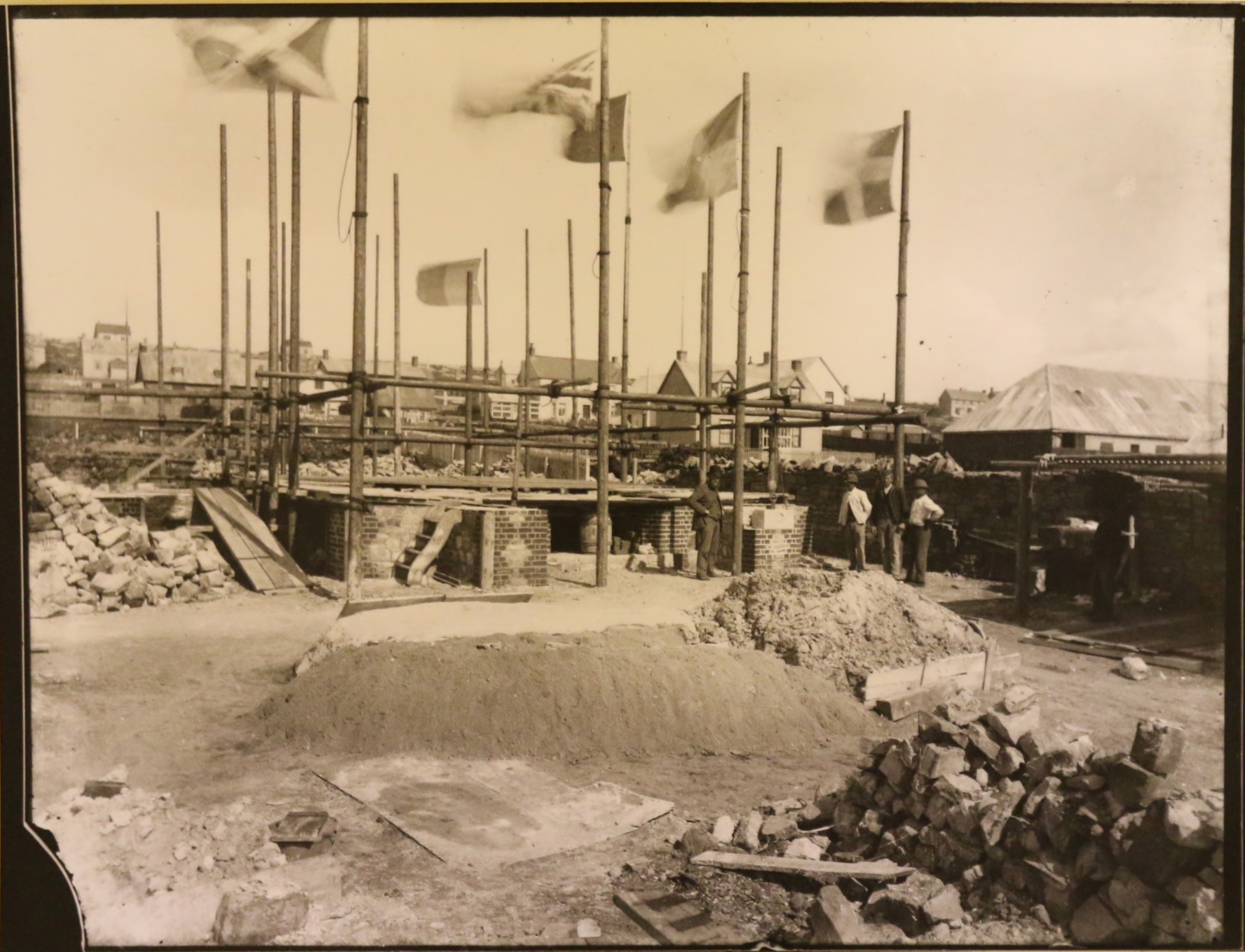
Foundations of Christ Church Cathedral c 1890
