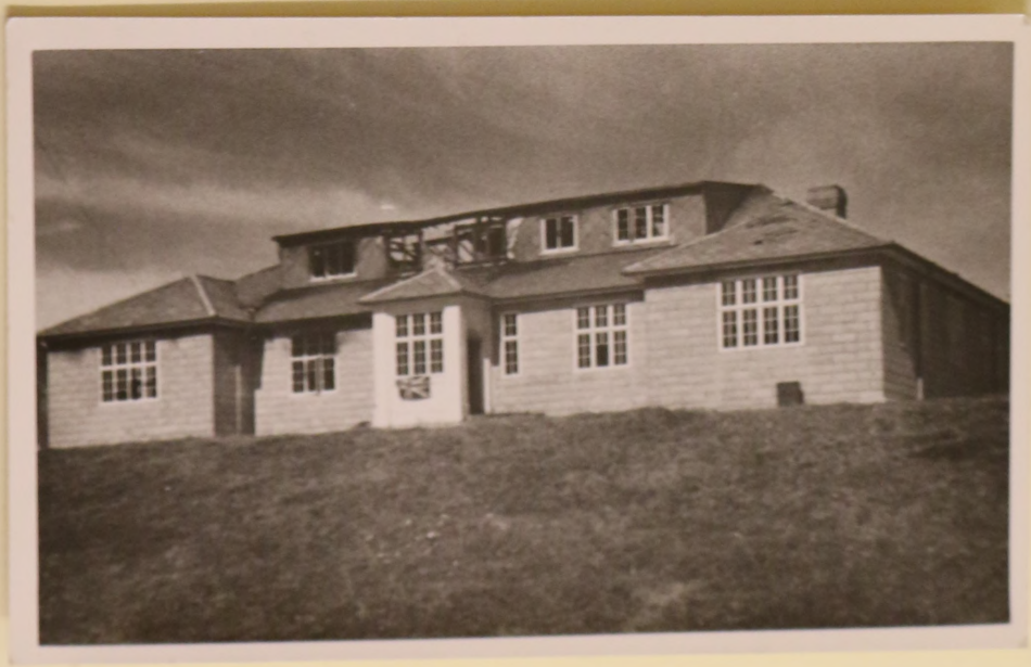
Secretariat after the fire of 9 March 1959
