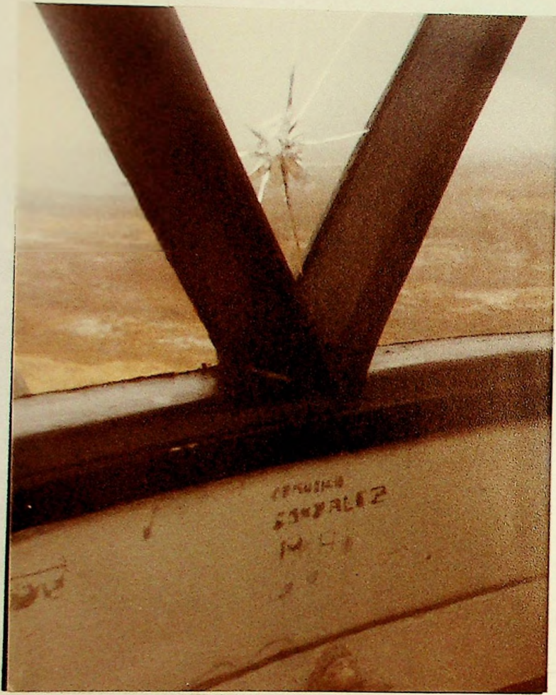
BULLET HOLE IN LANTERN GLAZING
