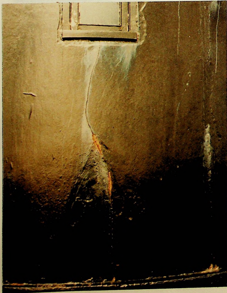
CRACK IN TOWER BASE
