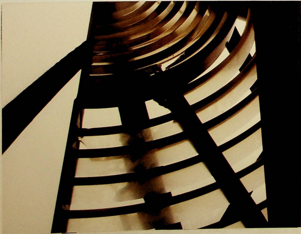
BROKEN PRISMS IN OPTIC
