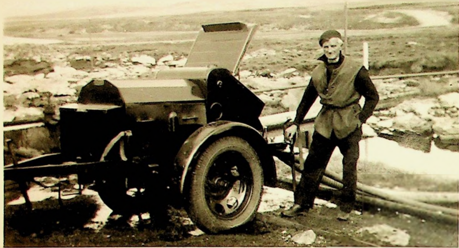
FIRE PUMP AT MOODY BROOK, NOVEMBER 1952
