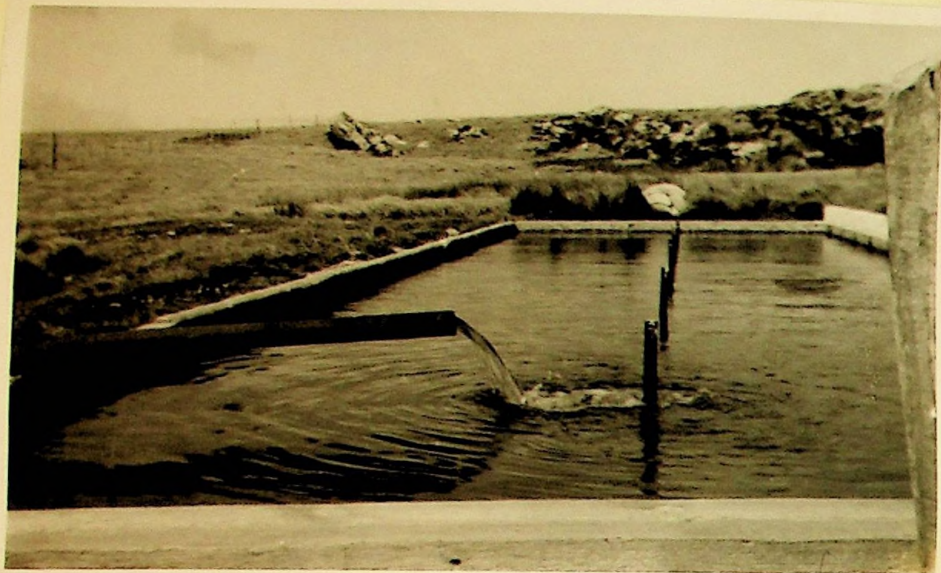
Flow from FIRE-PUMP DISCHARGING AT MT WILLIAM FILTERS
