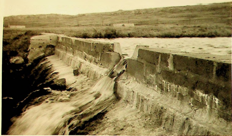
"V" NOTCH GAUGE ON TROUT-HATCHERY WEIR, MOODY BROOK
