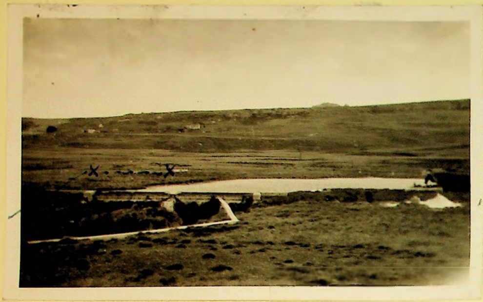
TROUT - HATCHERY WEIR AND POOL, MOODY BROOK. X = site for no used treatment plant
