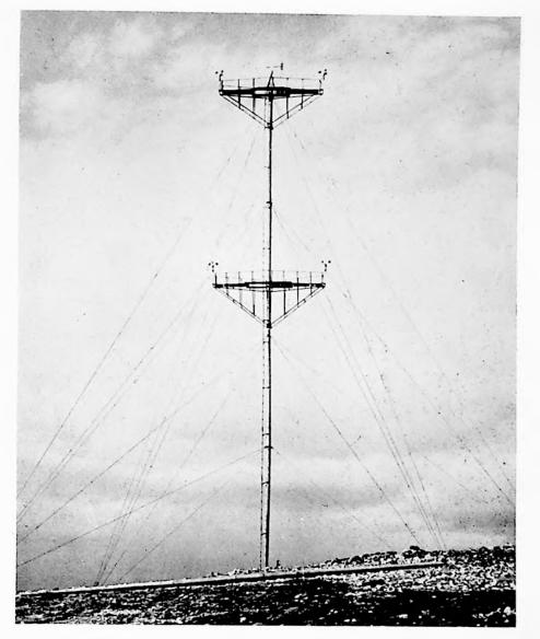
Fig. 5(a).-66-ft. tubular steel mast installation-Mynydd Anelog, North Wales.
