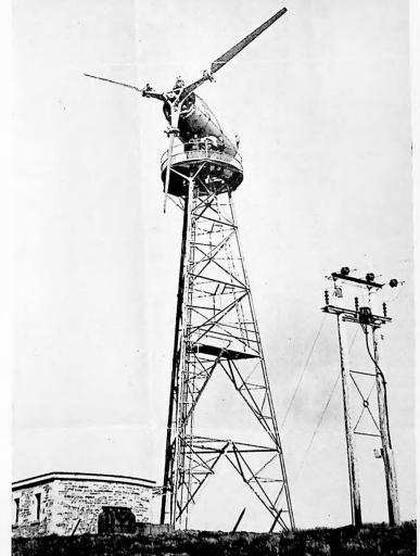
Fig. 1 The 100-kW generator on Costa Head consists basically of a triangular-section steel tower, a control room at the base of the tower, and a nacelle containing the step-up gearbox and generator. The generator output is transformed to 11 kV and fed into the Orkney mainiand distribution network through the overhead line.
