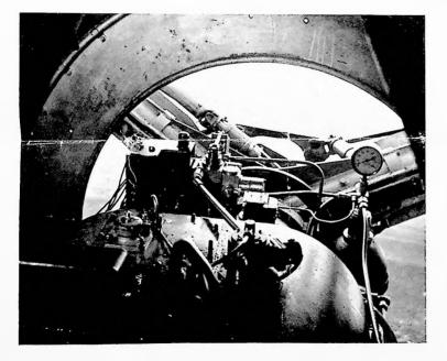
Fig. 5 The governor and inboard parts of the hub shown from inside the nacelle; one of the torque tubes which adjust blade pitch can be seen at the far end of the governor mechanism going off upwards and to the left
