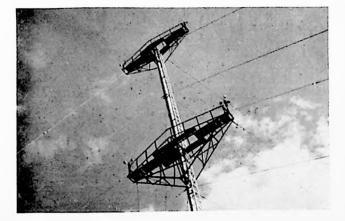
Fig. 5(b).--66-ft. mast at Anelog, showing guys and platform construction.
