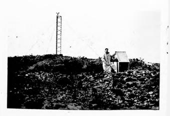
Fig. 4.—Coal-bunker housing recorder for 15-ft, lattice tower installation—St. Agnes Beacon, Cornwall.
