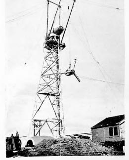
Fig. 6 A stage during construction, showing the hub and gearbox being lifted into position in the nacelle. The top half of the nacelle can be seen lying on the ground at the foot of the tower.
